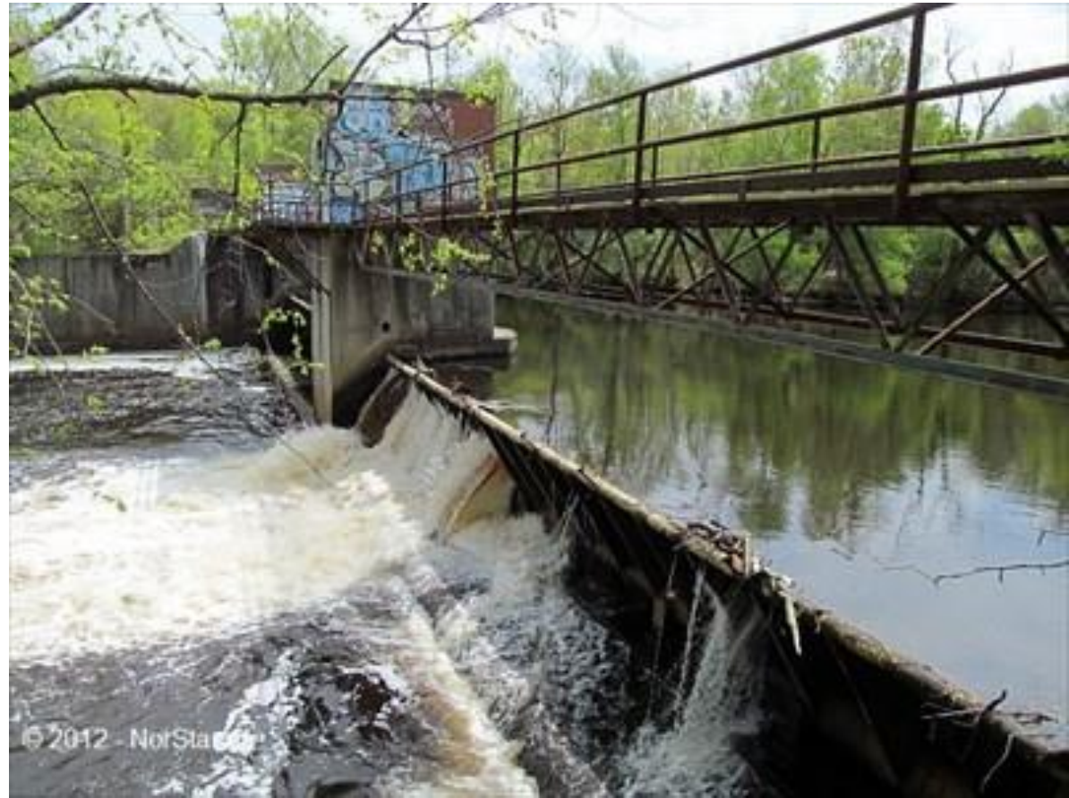
Tileston and Hollingsworth Dam – Boston
