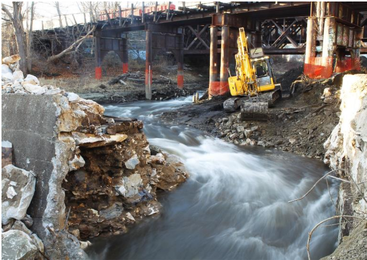
Tel-Electric Dam – Pittsfield photo DER
