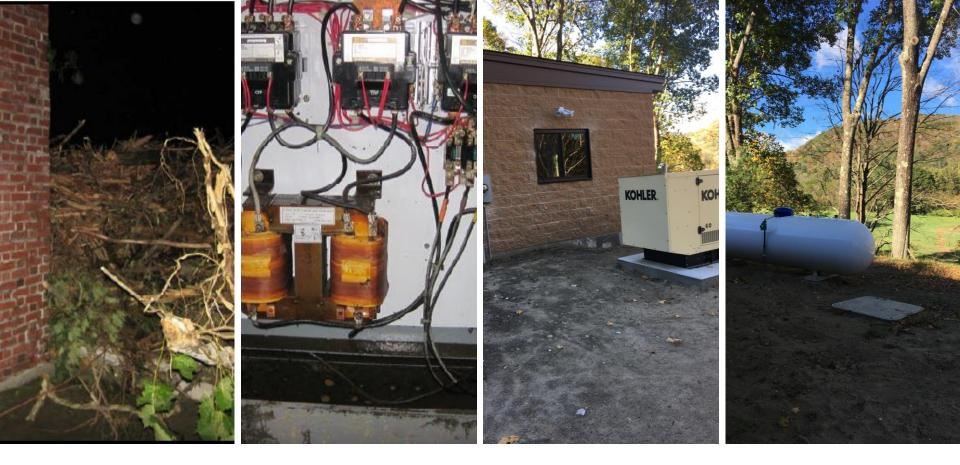
Pump Station Electrical Controls Relocated: Shelburne Falls Pump station electrical controls were relocated and a new generator was installed.
