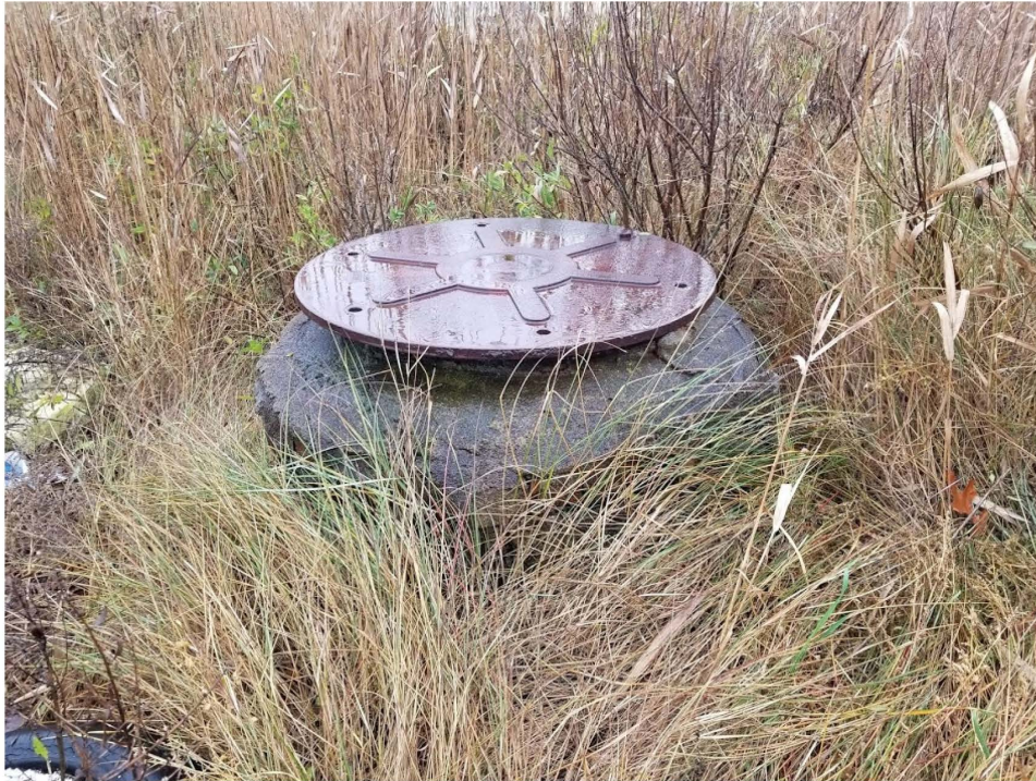
Figure 7: Fore River Sewer manholes: Town of Braintree/ MWRA designed to open and discharge sewage
