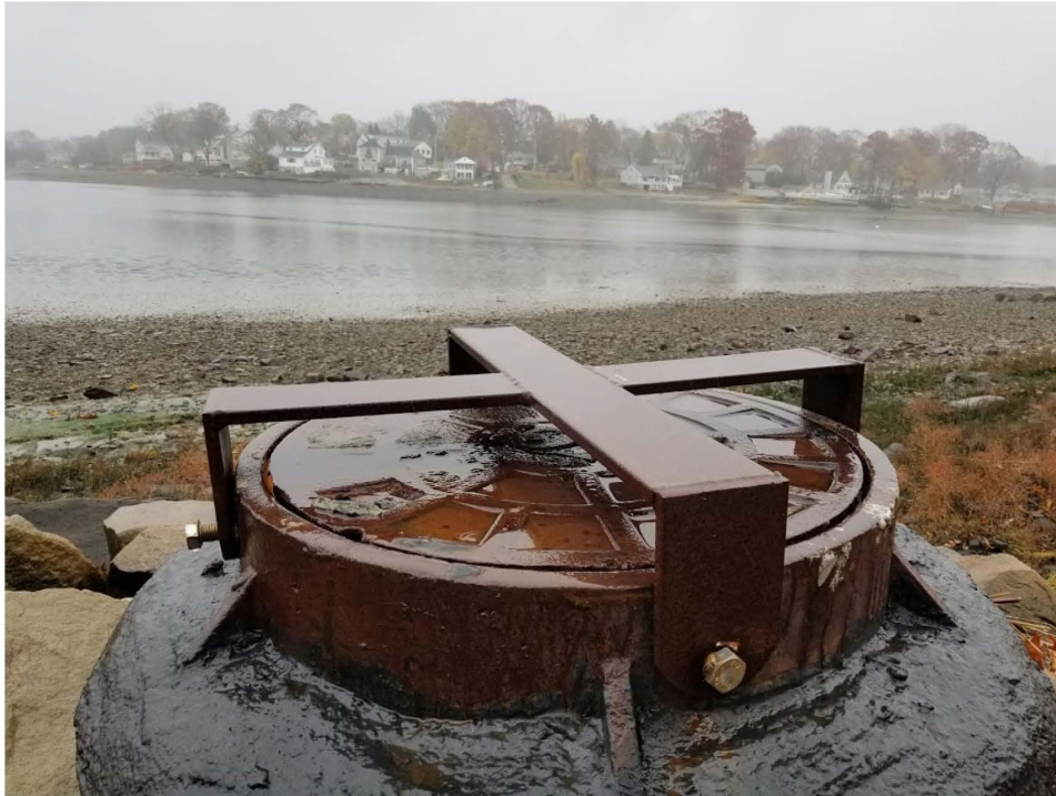
Figure 5: Fore River Sewer manholes:Town of Braintree/ MWRA designed to open and discharge sewage
