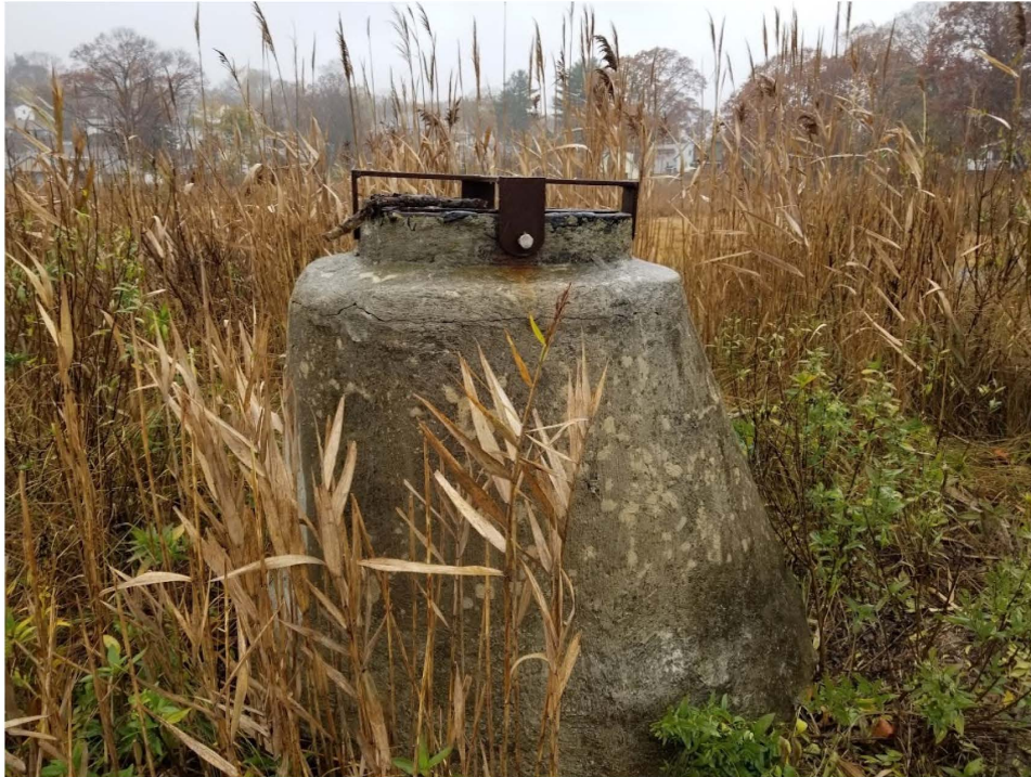
Figure 6: Fore River Sewer manholes: Town of Braintree/ MWRA designed to open and discharge sewage
