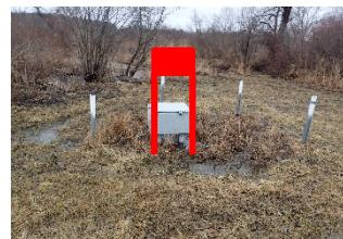
The well and its associated electrical equipment has been affected by beaver activity re-routing portions of the river and leading to potential flooding impacts on the power and control equipment adjacent to the well.
