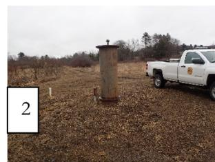
Raising the electrical junction box or relocating this box and installing watertight conduit would further protect this supply from not being available during flooding events.
