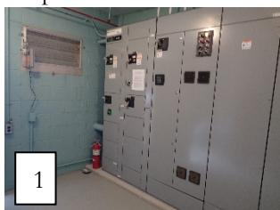
The floor elevation for the wellhouse is approximately 634.6 which is over 7 feet above the 100 year flood elevation. The only electrical equipment which is susceptible to flooding is the MCC which rest on a housekeeping pad only 4 inches above the floor (Photo 1) and an electrical control cabinet which is 33 inches above the floor.
