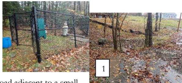
stream that flows past it. The ground elevation in the area is 772.8 based on LIDAR information. The pump station is a wetwell submersible station with an electrical power/control panel, a ventilation system and it is surrounded by fencing for security.
