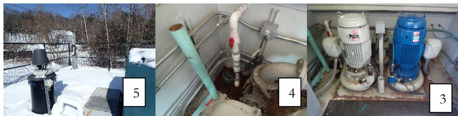
components below grade against flooding. Further, the main service outside should be protected against flooding. This can be accomplished by installing walls around the facility or by upgrading the facility and elevating critical components above grade in a new structure.
