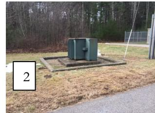
Just outside the building is the main power transformer for the site which rests on the ground (Photo 2). This would be adversely affected if the site was flooded. This should be raised to protect it against potential flooding.
