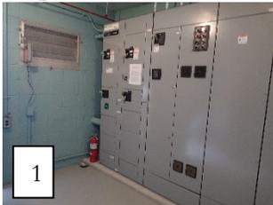
The floor elevation for the wellhouse is approximately 634.6 which is over 7 feet above the 100 year flood elevation. The only electrical equipment which is susceptible to flooding is the MCC which rest on a housekeeping pad only 4 inches
