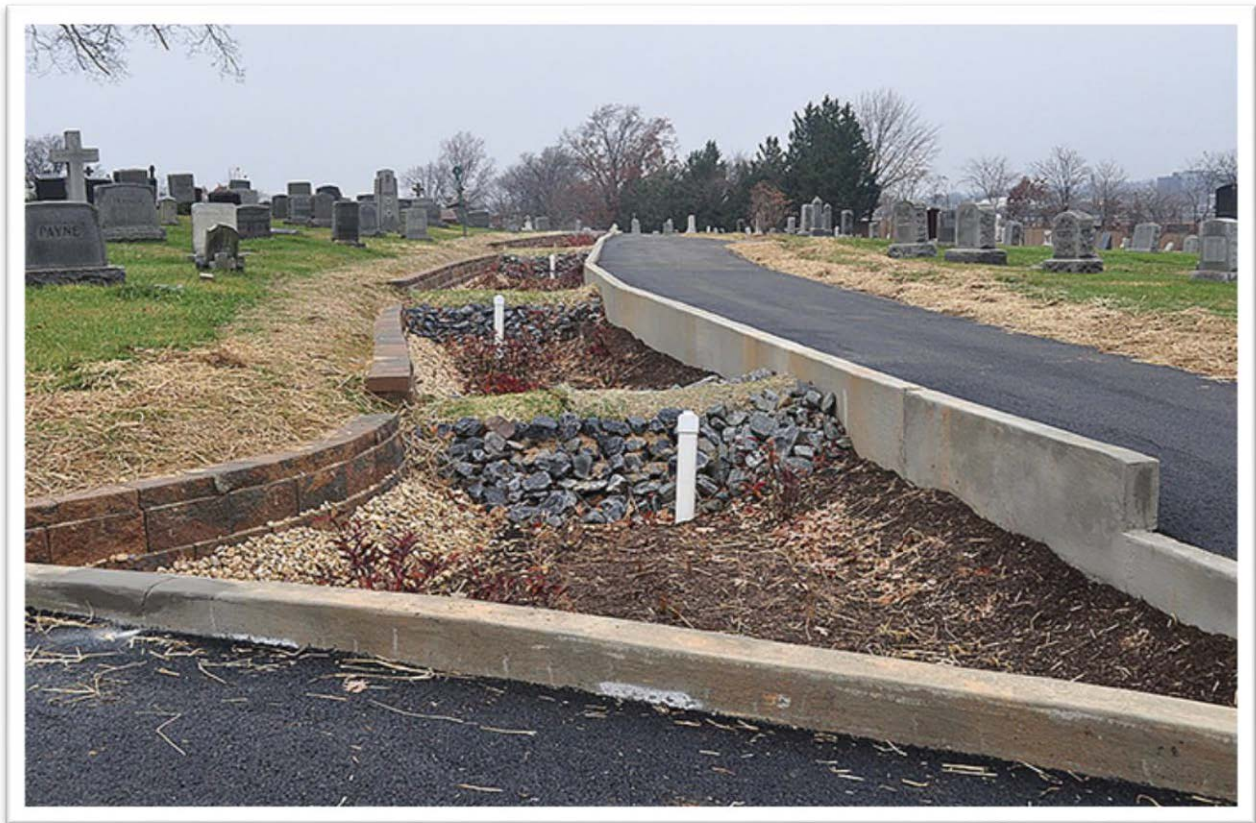
Figure 33 Bio-retention area installed at a narrowed drive at Mount Olive Cemetery, Washington, DC.
