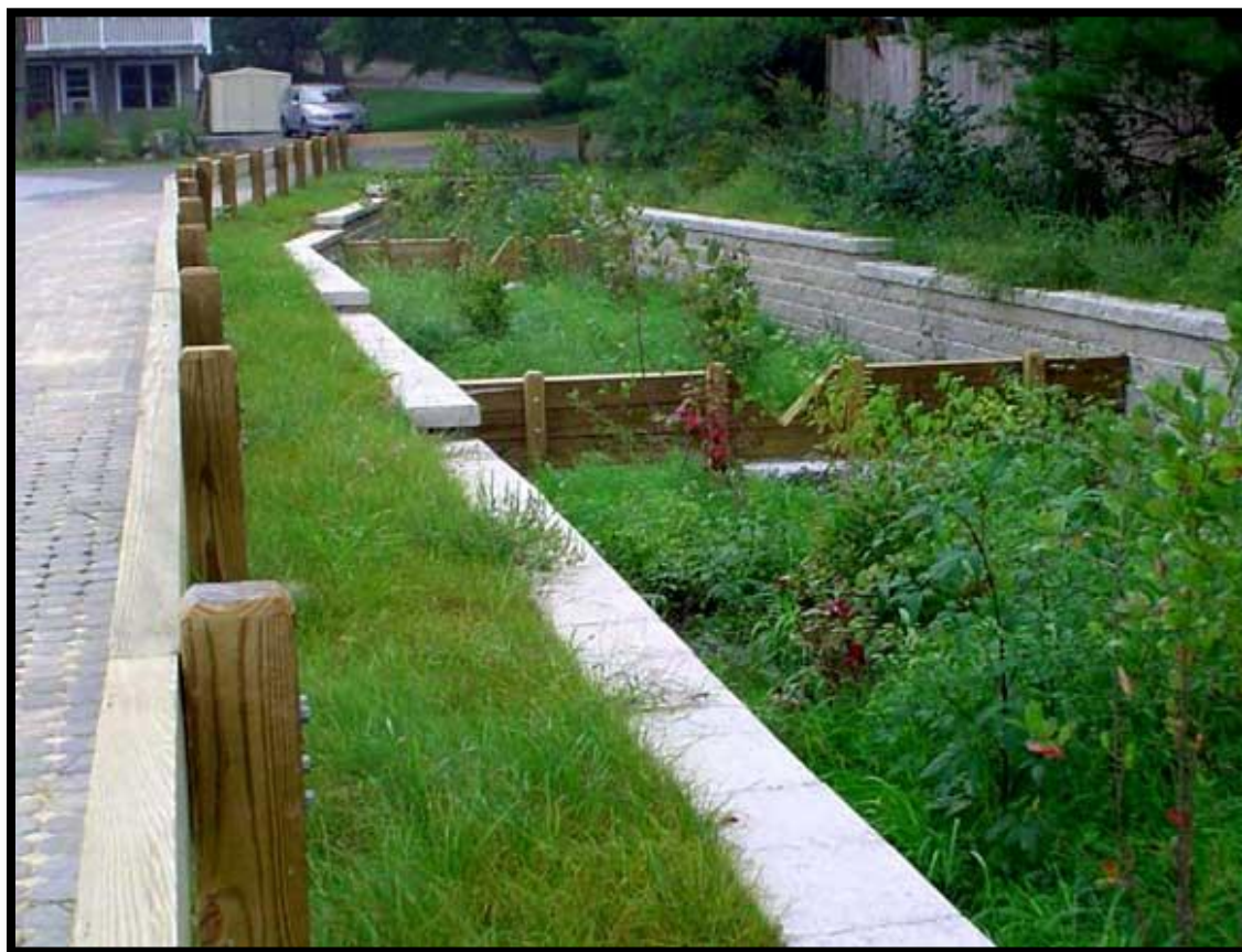
Figure 44 Vegetated swale with erosion control walls, Long Pond, Littleton, MA.
