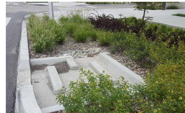
Image 4: Example of an established bioretention basin with a concrete curb cut and concrete pretreatment structure to remove sediment before runoff enters the planted portion of the basin.
