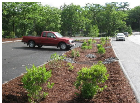
Image 3: Example of a parking lot with bioretention and diagram of a bioretention basin. Image source: MA Clean Water Toolkit.
