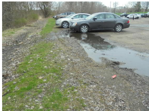
Image 1: Existing swale and runoff forming concentrated flow over the embankment into the swale.
