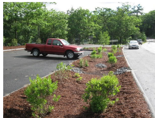
Image 3: Example of a parking lot with bioretention and diagram of a bioretention basin. Image source: MA
