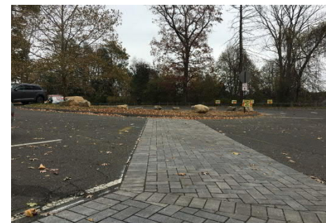
Image 4: Typical installation of a permeable paver walkway in a municipal parking lot. Image Source: Fuss & O'Neill.
