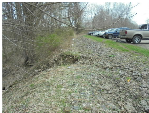
Image 2: Severe erosion at the outlet of the existing swale.
