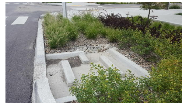
Image 3: Example of an established bioretention basin with a concrete curb cut and pretreatment structure to remove sediment before runoff enters the planted portion of the basin.
