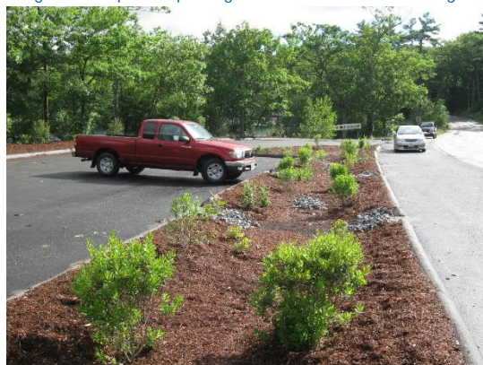
Image 1: Example of a parking lot with bioretention and diagram of a bioretention basin. Image source: MA Clean Water Toolkit.
