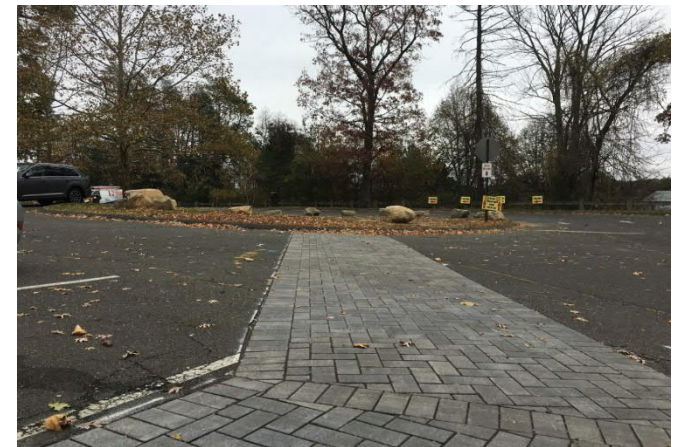
Image 4: Typical installation of permeable paver walkway in a municipal parking lot. Image Source: Fuss & O'Neill.
