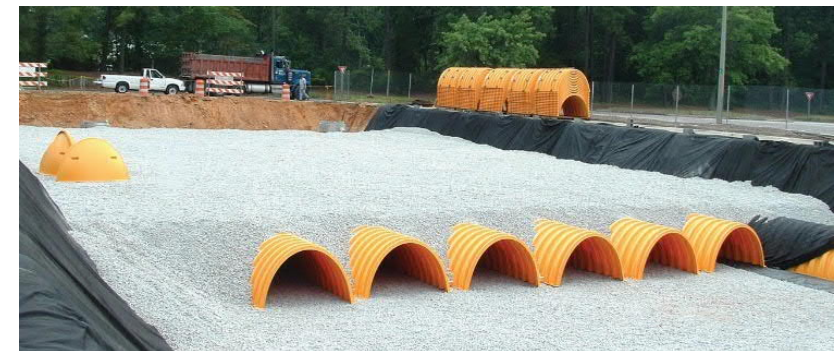
Image 3: Typical installation of underground infiltration system below an existing parking lot. Image source: stormtech.com
