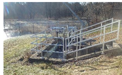
UV Disinfection System at the Discharge of the Wastewater Treatment Facility
