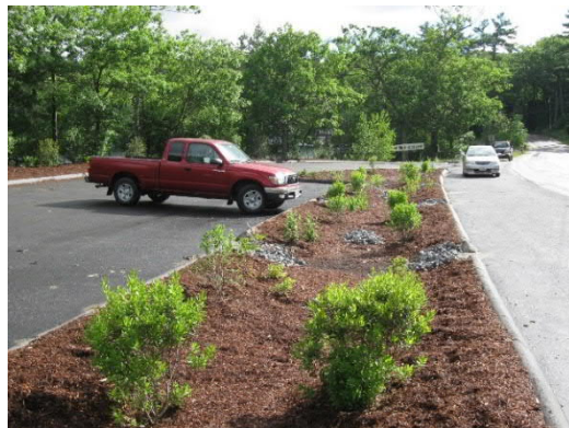
Image 2: Example of a parking lot with bioretention and diagram of a bioretention basin. Image source: MA Clean Water Toolkit.
