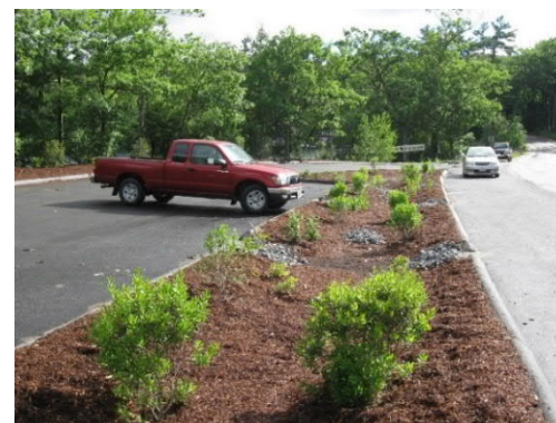
Image 3: Example of a parking lot with bioretention and diagram of a bioretention basin. Image source: MA Clean Water Toolkit.
