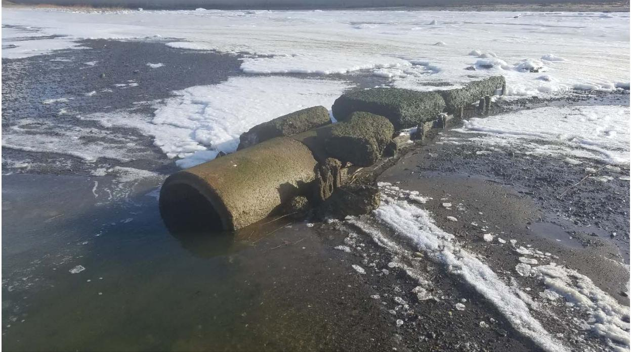
Photo 1 – Outfall at the point of discharge at Mean Low Water with broken up concrete and separated pipes.
