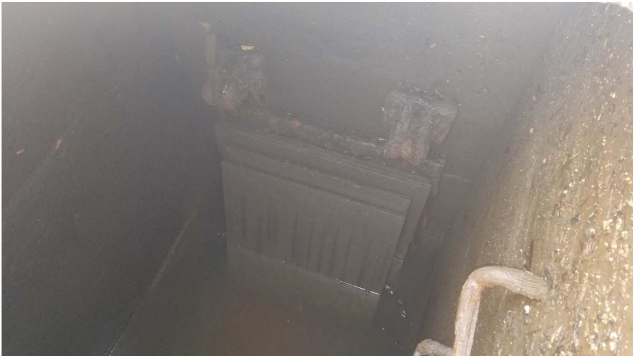
Photo 2 – Inside the tide gate structure looking at the corroded tide gate on the downstream side.
