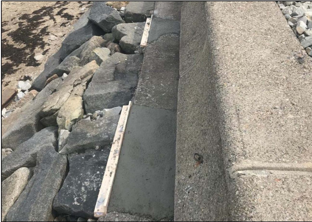
Leveling slab repaired at pre-cast seawall
