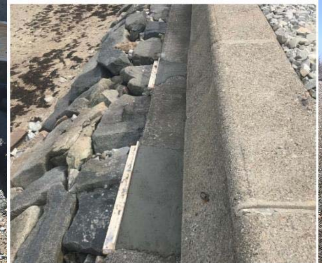
Leveling slab repaired at seawall along Shelton Rd.
