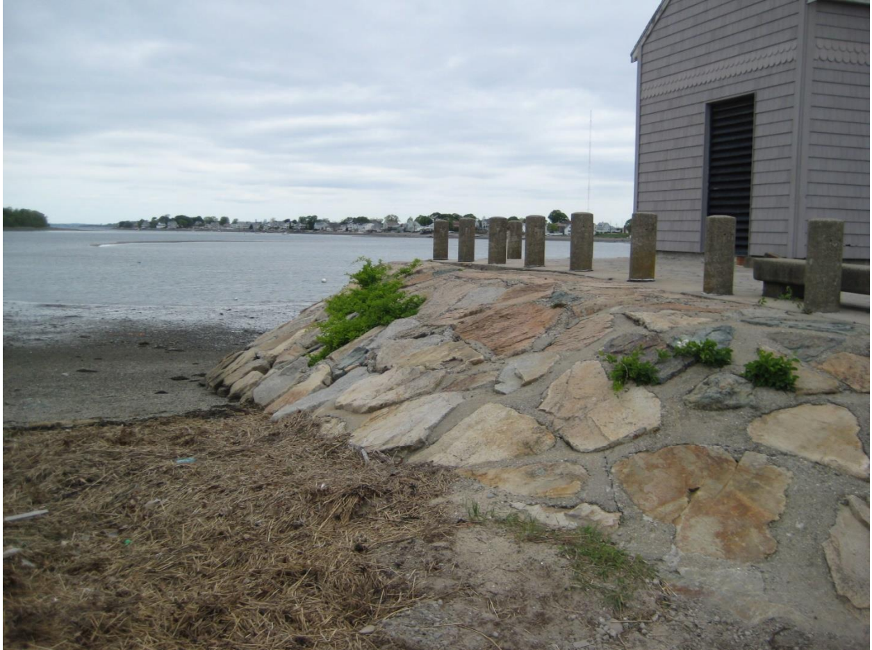
Figure 3. The pump station is situated on a pile-supported concrete slab fronted by a grouted armor stone revetment. The tide line is visible on the left side of this photo.
