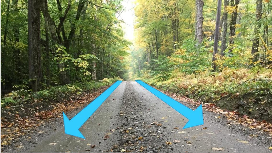
*Entrenched roads trap drainage on the roadway. As this drainage flows downhill, it generally increases in both volume and velocity, resulting in the erosion of road material.*
