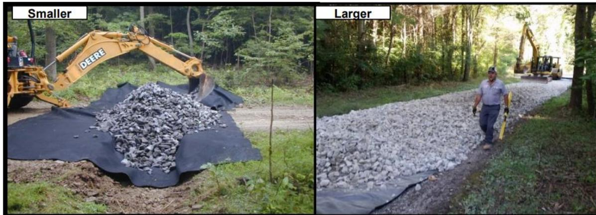
Smaller and Larger French Mattresses During Construction (Source: Penn State Center for Dirt and Gravel Road Studies)<sup>18</sup>
