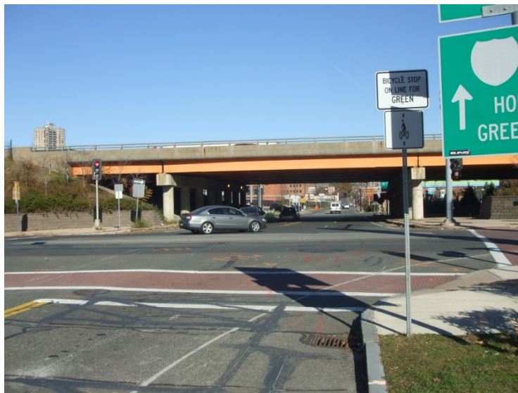
Figure 2-43: West Columbus Avenue (Hall of Fame Avenue) at Union Street – Pavement marking symbols and interstate shield at the eastbound approach are worn.
