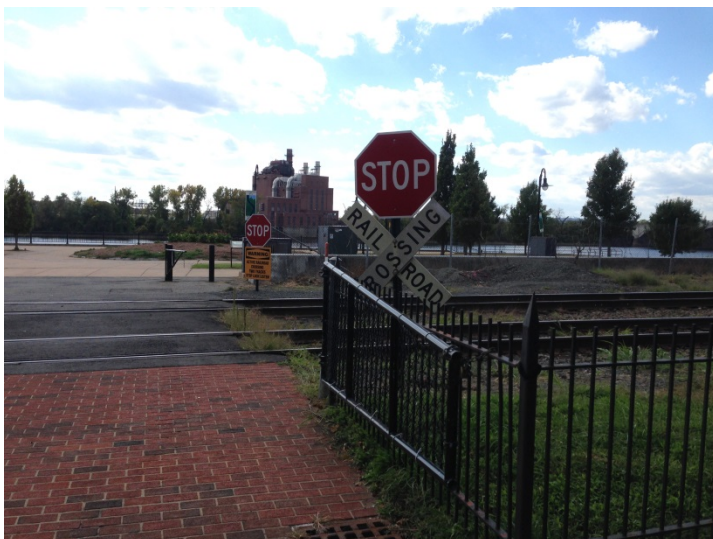
Figure 2-39: Passive At-Grade Highway-Rail Crossing at Riverfront Park
