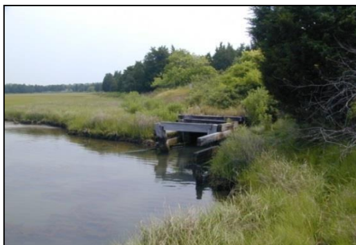
Figure 8. Existing Non-Functioning Culvert beneath Ray Peck Drive
