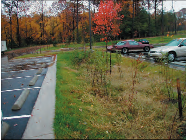
FIGURE 29. A biofiltration area in a parking lot.
