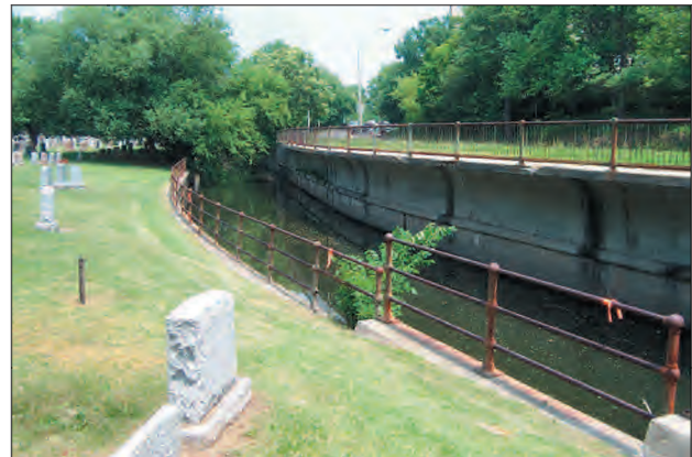
FIGURE 61. On the east side, a concrete retaining wall with a cantilevered sidewalk defines the brook's edge in the Parkway section between Henderson bridge and Broadway.
