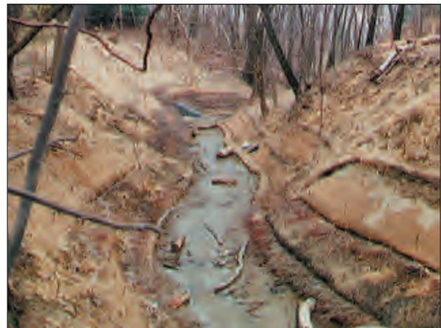
FIGURE 24. This stream channel is being restored using bioengineering techniques. These techniques, originally developed in Europe, combine mainly natural materials such as native plants, coconut fiber mats, and rock. They have proven very successful in restoring natural systems.
