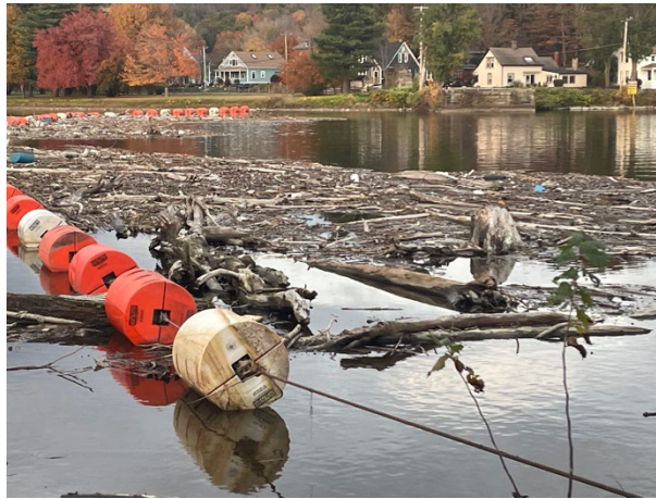
Figure 8: Trash and debris behind the TFD boat barrier. Kelsey Wentling, Oct. 2023
