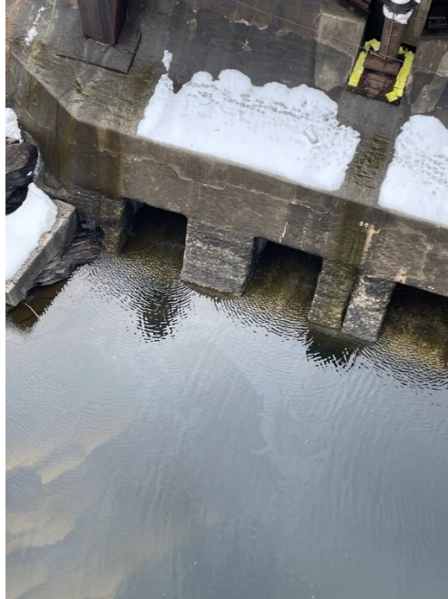
Figure 6: CRC photo taken March 17, 2023: Oil Sheen on the Connecticut River below Turners Falls Dam
