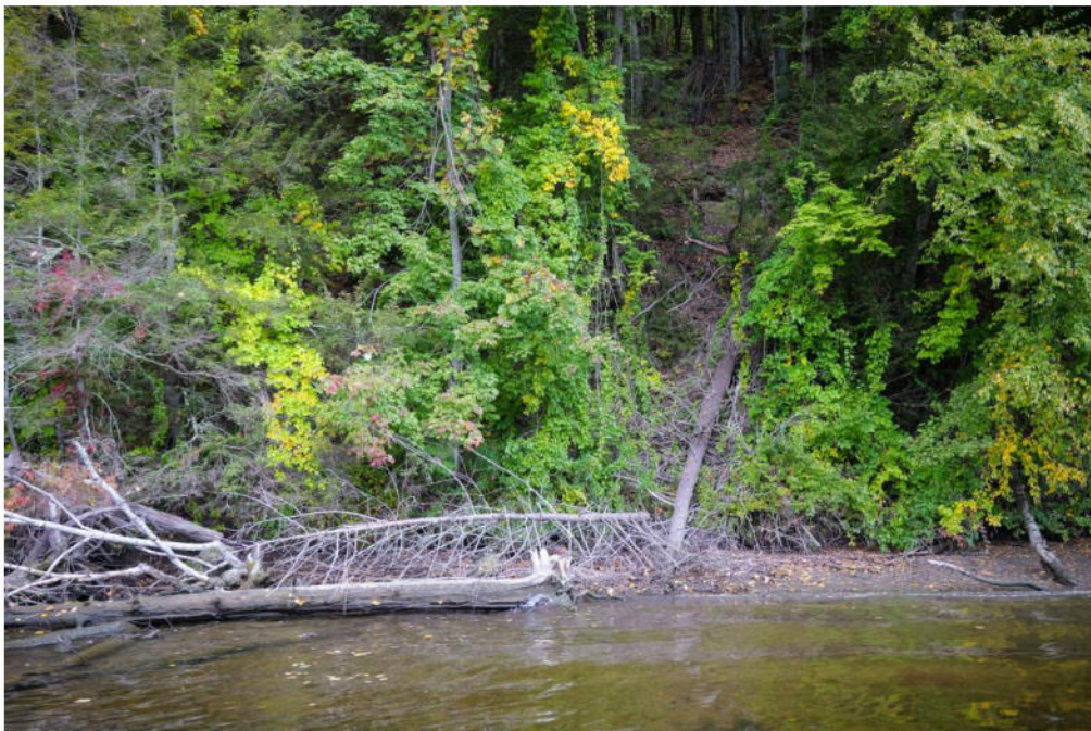
2024 CRC Site 2 (12): Landslide
