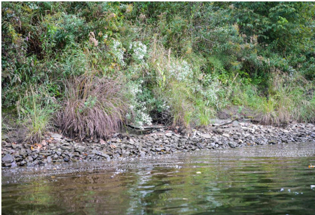
2024 CRC Site 12 (5) : Previous restoration site where vegetation is unable to grow in the water fluctuation zone
