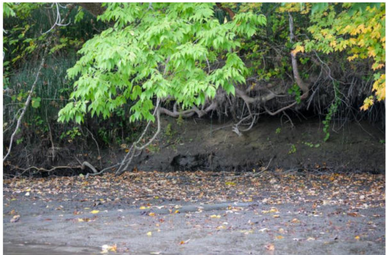
2024 CRC Site 9 (21) Close-up of eroded area
