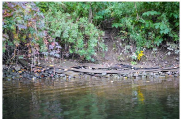
2024 CRC Site 8 (20) Loose fabric and erosion uphill
