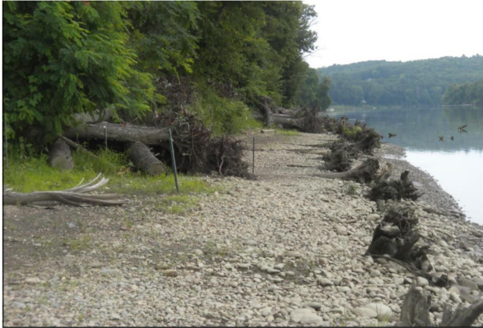
2024 (March): Looking north on Bathory/Gallagher site from the access road Stone and dirt has been eroded and logs with root wads have become exposed and dislodged since the 2013 restoration project installation.
