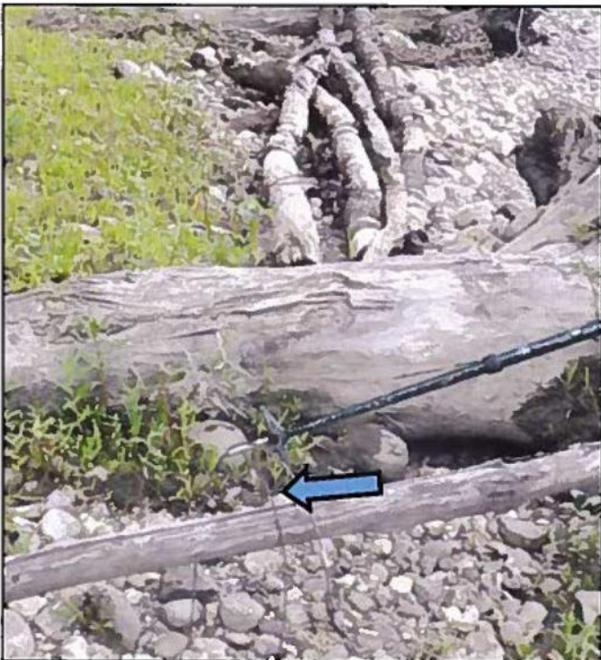
Loose anchor wire and missing log
