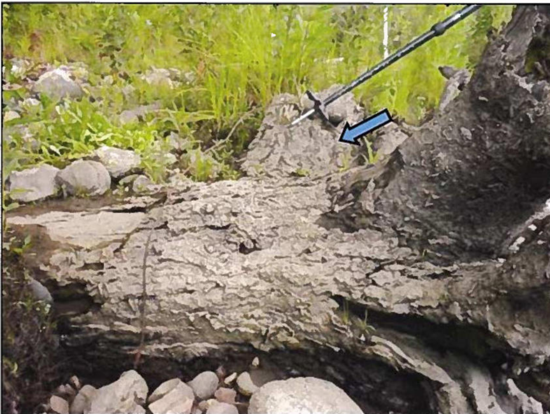
Loose anchor wire
