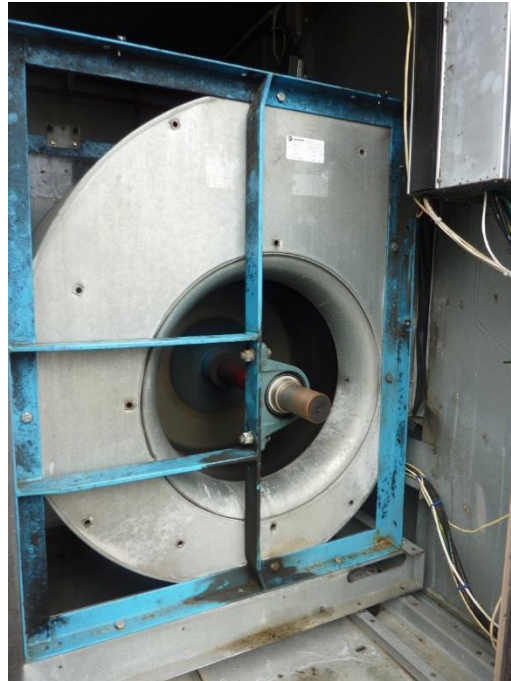
Photo 1 – Suspect visual mold on RTU fan assembly
