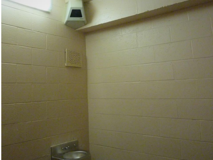
Photo 4 – Holding cell with modified exhaust grille
