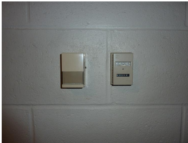
Photo 6 – Dual Pneumatic Thermostats Serving a Typical Zone
