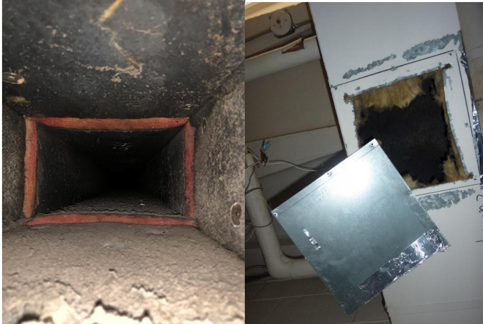
Photos 2 and 3 – Fiberglass duct liner and loose edges at test panel
