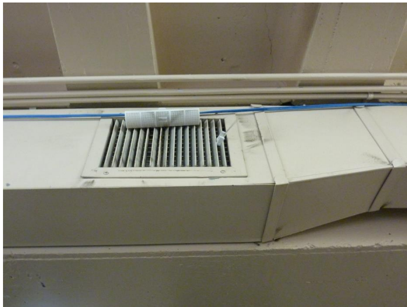
Photo 5 – Supply diffuser in corridor outside holding cells
