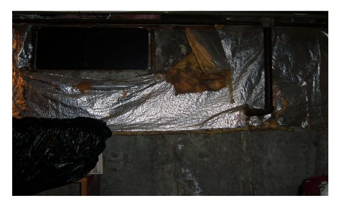
200-1 Development, Normandy Road -Heating Duct Insulation Peeling from Basement Ceiling
