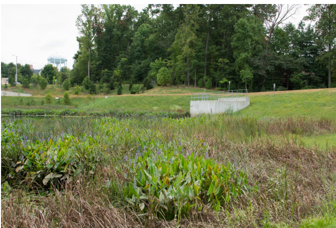
Figure 4: View looking north across project site
