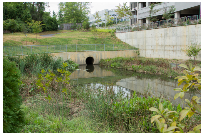
Figure 3: View looking west across project site showing outfall
