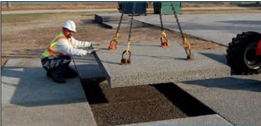
Concept for modular pre-cast porous pavement slabs and subsurface storage at public school parking lot (image source: Stormcrete)
