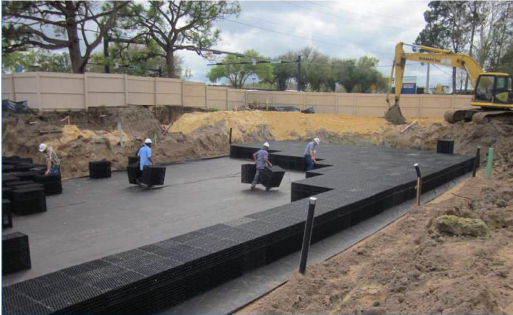
Figure 5-2: Typical R-Tank Installation (Source: ACF Environmental)
