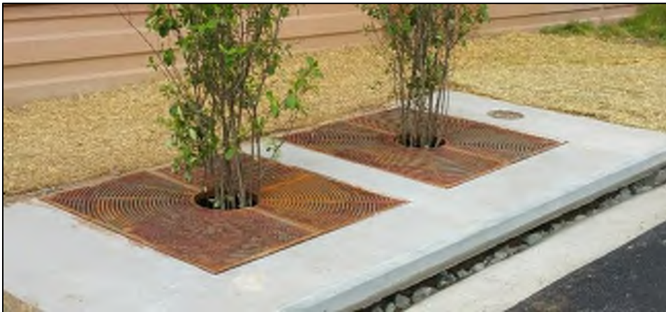
Concept for Filterra modular stormwater tree pit to reduce spot erosion near Tufts Park east entrance (images source: Contech)
