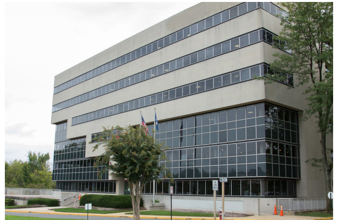
Figure 5: Front and west side of building
