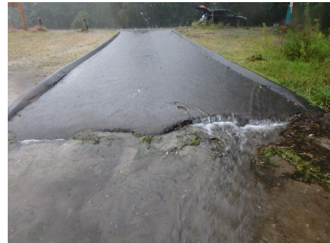
Photo 2. Sheet flow runoff from River Street along the former boat launch into Forest Lake
