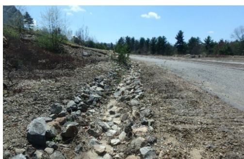
Photo 1. Example of roadside ditch where vegetation would provide additional pollutant attenuation.
