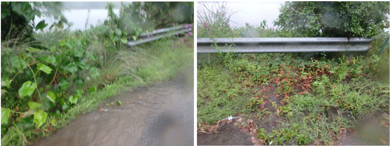
Photo 3. Sheet flow from River Street discharging to Forest Lake west of the beach
