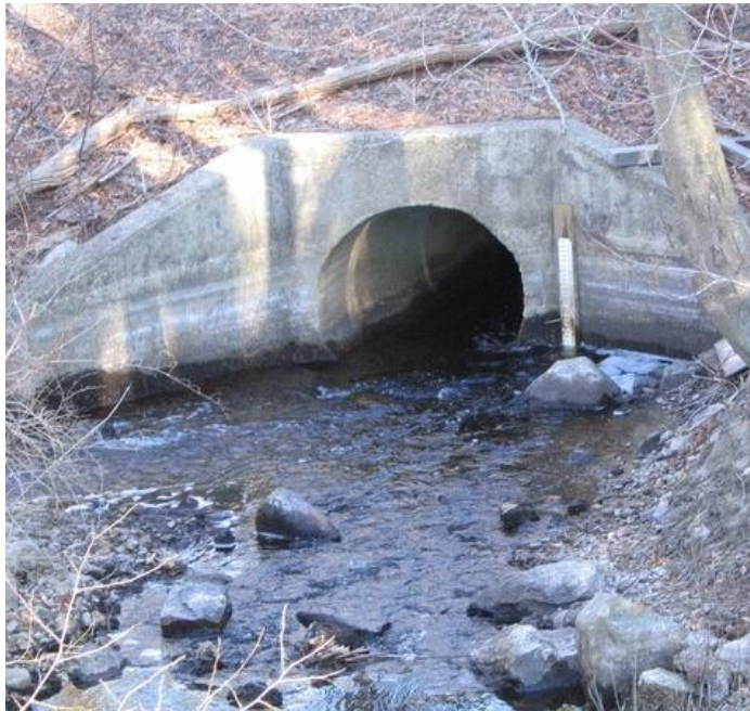
Upstream face of Lake Street culvert with RIFLS staff gage
