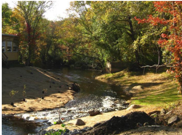
Site of Former Wapping Road Dam (looking downstream)
