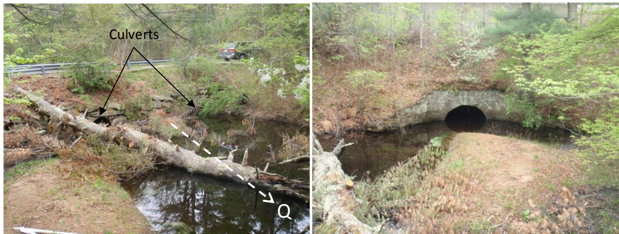
Grove Street Culverts
