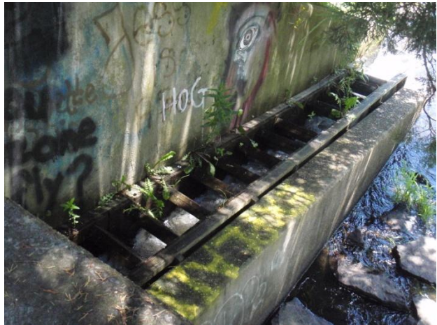
Furnace Pond Dam fish ladder, looking downstream
