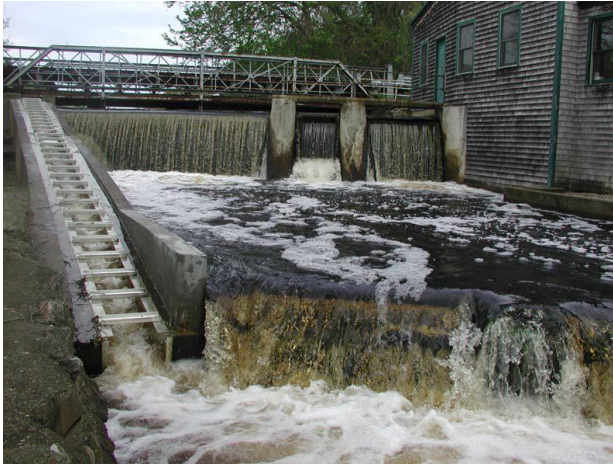
Elm Street Dam and Fish Ladder
