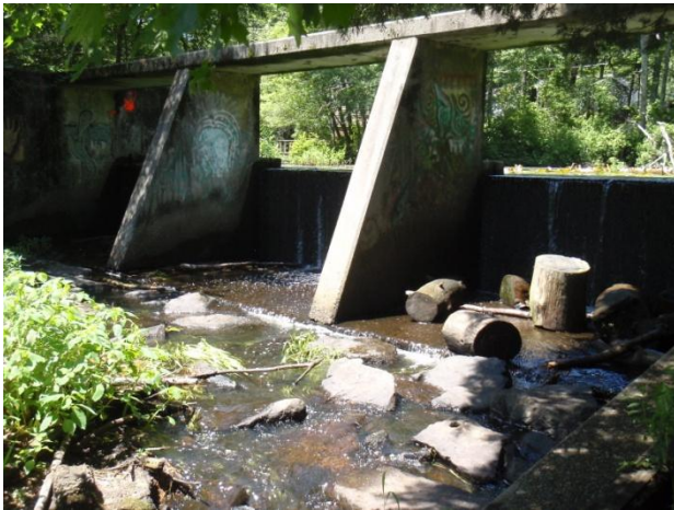
Furnace Pond Dam, looking upstream
