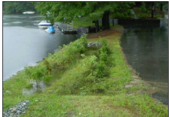
Lakeside rain garden providing storage during a rain storm (Lake Shirley, Lunenburg, MA).
