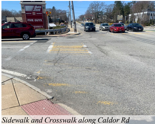
Route 9/Shoppers World Drive Intersection, missing pedestrian signals and accessibility infrastructure
