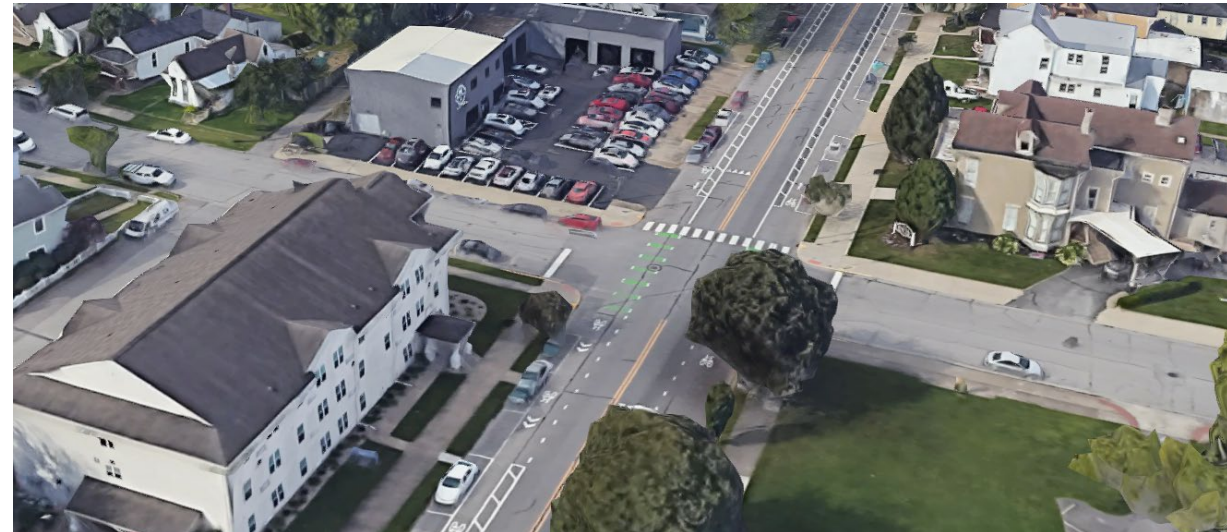
East Spring Street Two-Way Restoration, New Albany, IN
