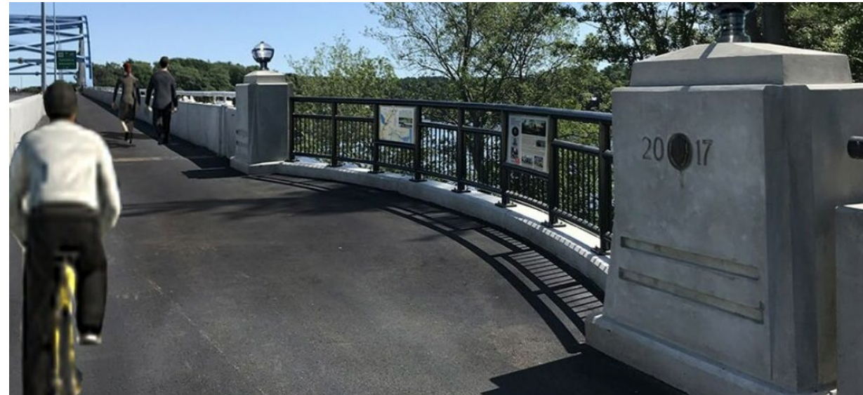
Protected Shared Use Path along Whittier Bridge in Amesbury, MA (Source: MassDOT)
