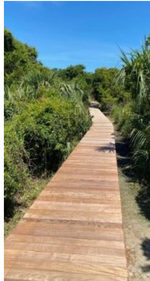
Shared Use Boardwalk
