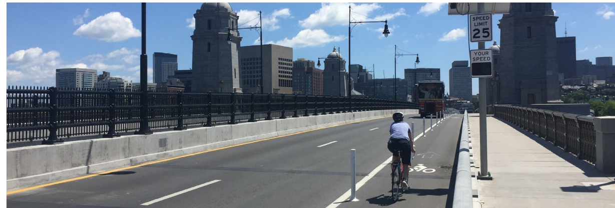
Dedicated Bicycle Lane and Protected Sidewalk along Longfellow Bridge in Boston, MA
