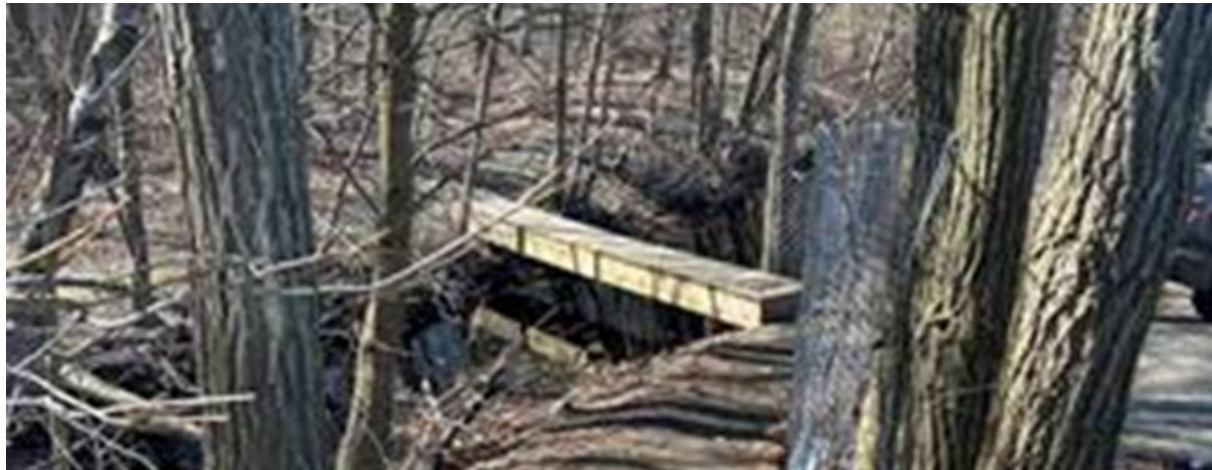
The Existing Connection between Travis Road and Sherwood Plaza
