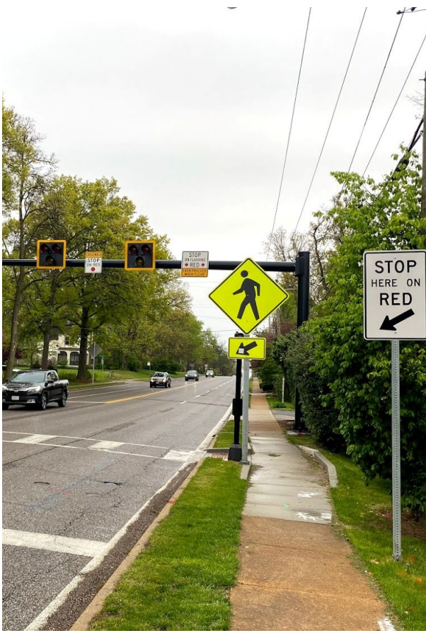
HAWK Signalization & Protected Sidewalk Kirkwood, MO
