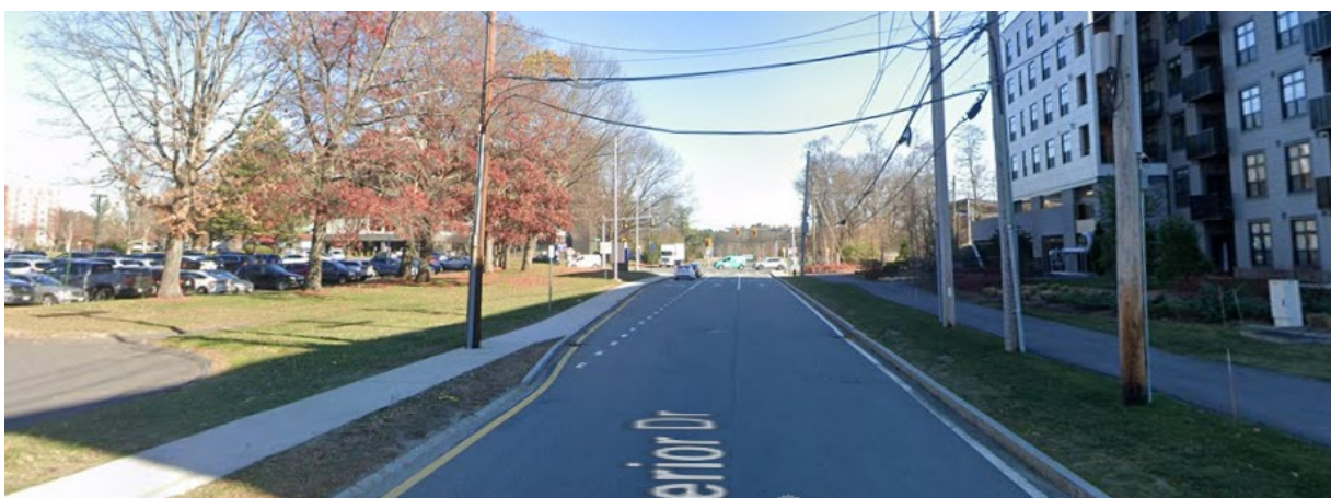
The Current Conditions along Speen Street and Superior Drive – sidewalks abruptly end and no dedicated bicycle facility exists.
