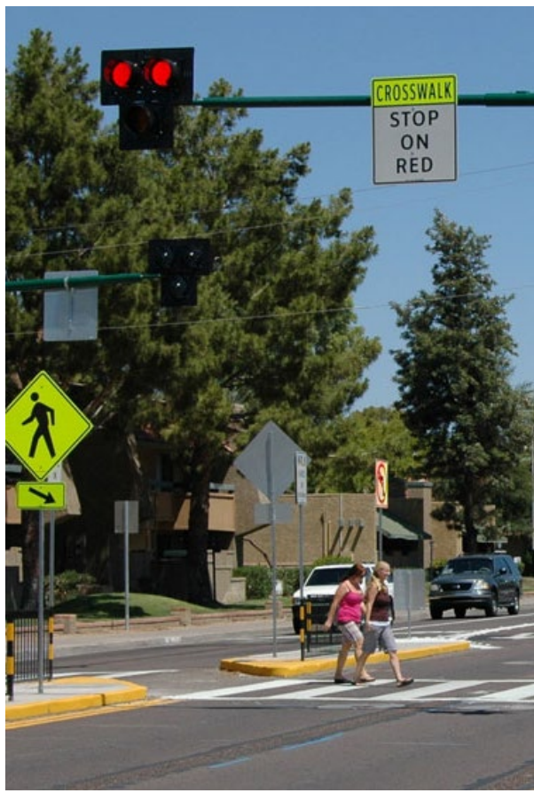
HAWK Signals Arizona Department of Transportation
