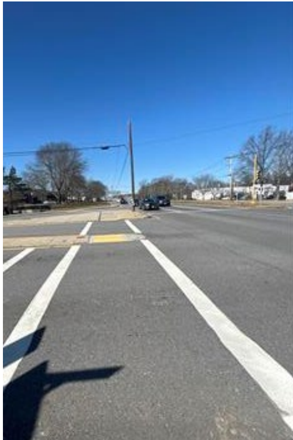
Missing Pedestrian Signals at the Route 9 and Sherwood Plaza Entrance
