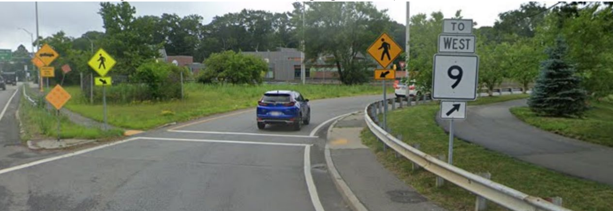
The Current Route 9/Speen St Intersection- guardrail blocking sidewalk connection to shared use path
