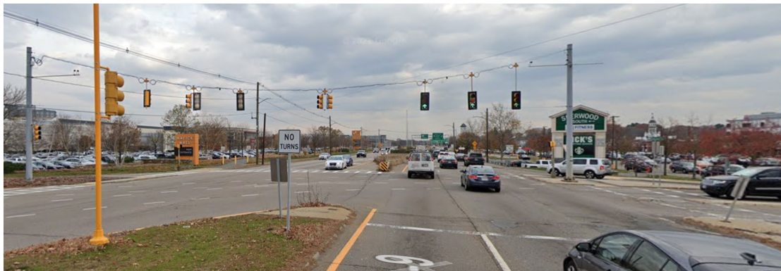
The Existing Conditions at the Route 9/Dean Road/Natick Mall Road Intersection- long crosswalks and missing pedestrian signal
