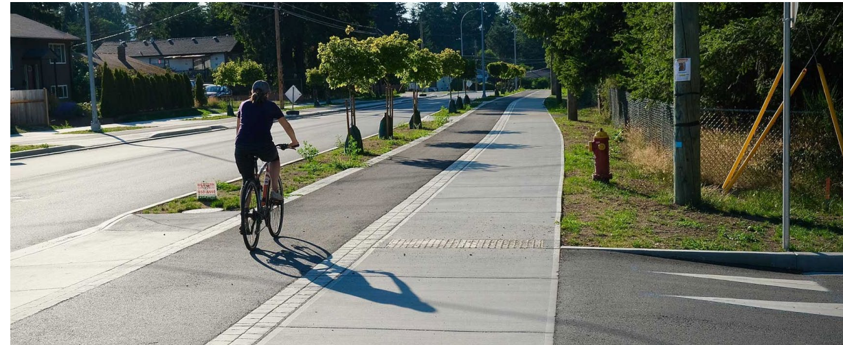
Dedicated Bike Lane and Sidewalk along Roadway: Small Town and Rural Design Guide
