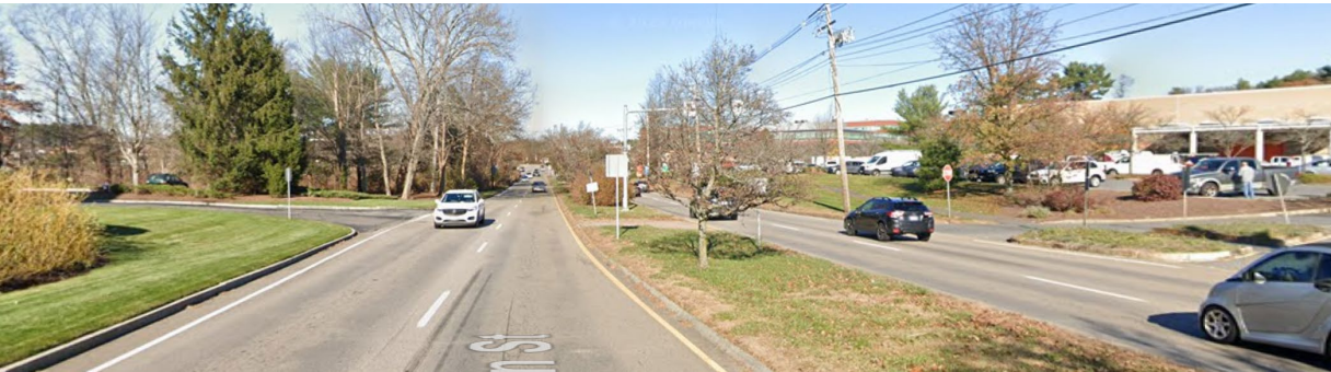
The Current Conditions of Speen Street between Route 30 and Nouvelle Way
