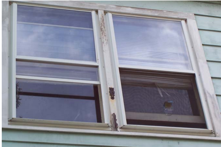
705-1 Development, 66-68 West River Street, Orange Hole in Screen and Rotted Wood around Window
