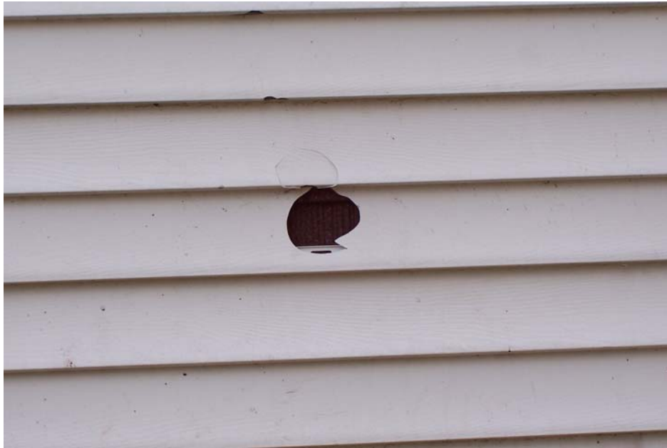
705-1 Development, 36C Congress Street, Orange Large Hole in Siding
