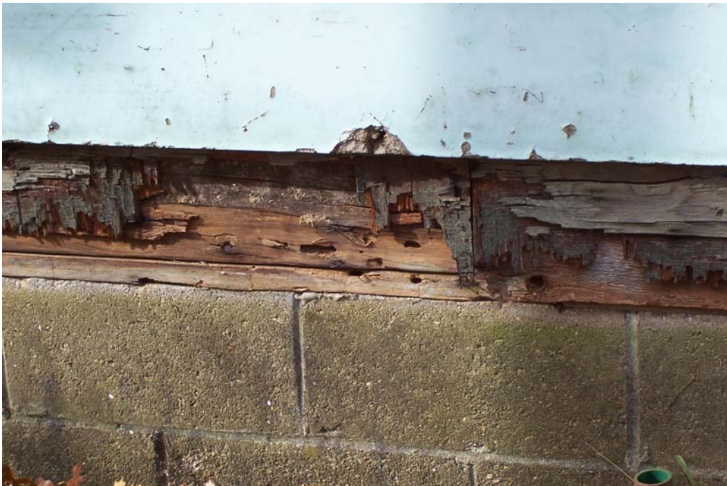
705-1 Development, 66-68 West River Street, Orange Insect Damage and Missing Wood Trim
