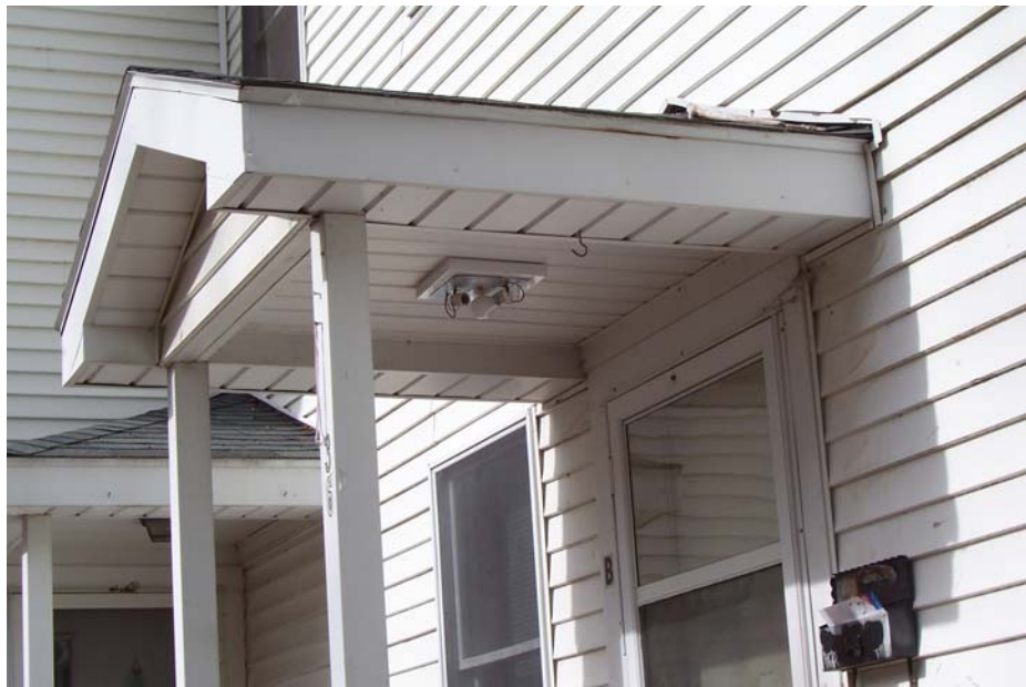
705-1 Development, 36C Congress Street, Orange Missing Light Bulb and Fixture Cover
