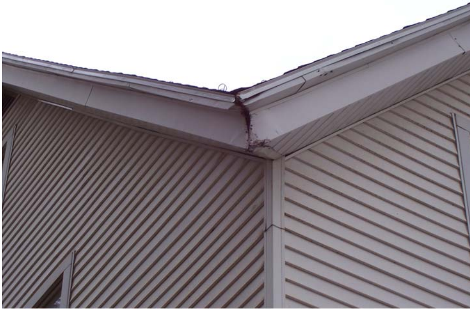
705-1 Development, 66-68 West River Street, Orange Siding Coming off and Rotted Window Trim
