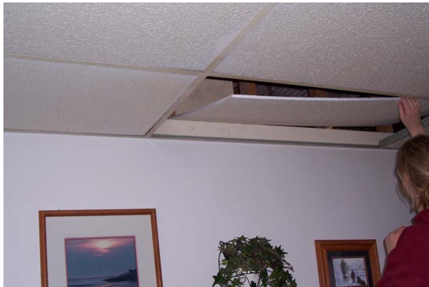
705-1 Development, 73 South Street, Bernardston Original Ceiling Falling Apart, Causing New Dropped Ceiling to Fall
