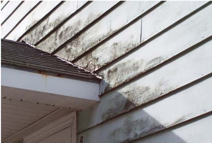
705-1 Development, 66-68 West River Street, Orange Siding Disintegrating above Entry Door
