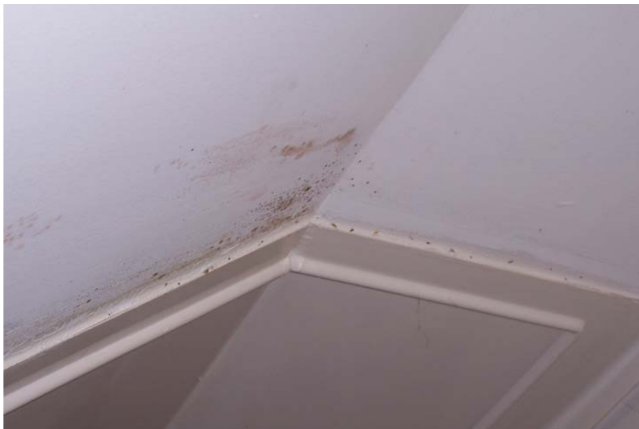
705-1 Development, 36C Congress Street, Orange Mold on Ceiling above Shower Stall
