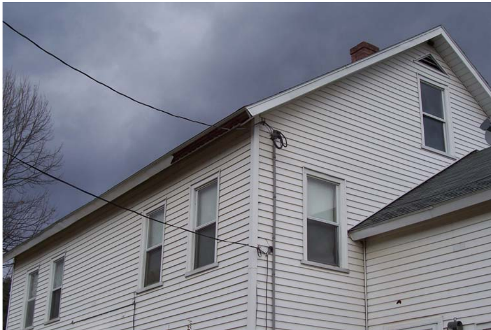
705-1 Development, 25 Main Street, Charlemont Vinyl Facing on Trim Board Missing
