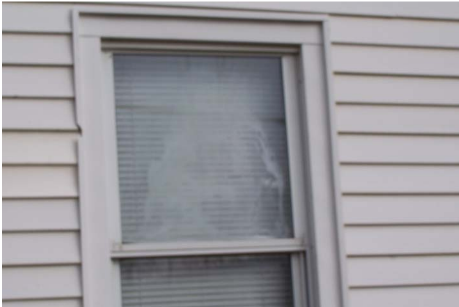
705-1 Development, 25 Main Street, Charlemont Vinyl Facing on Trim Board Missing
