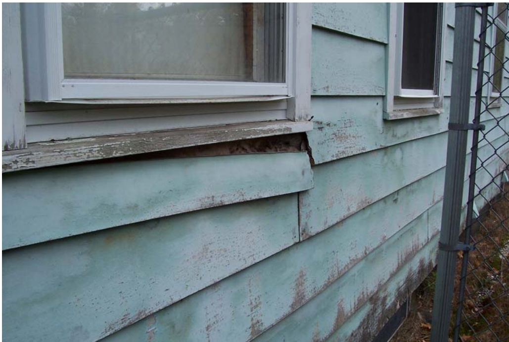
705-1 Development, 66-68 West River Street, Orange Siding Coming off and Rotted Window Trim
