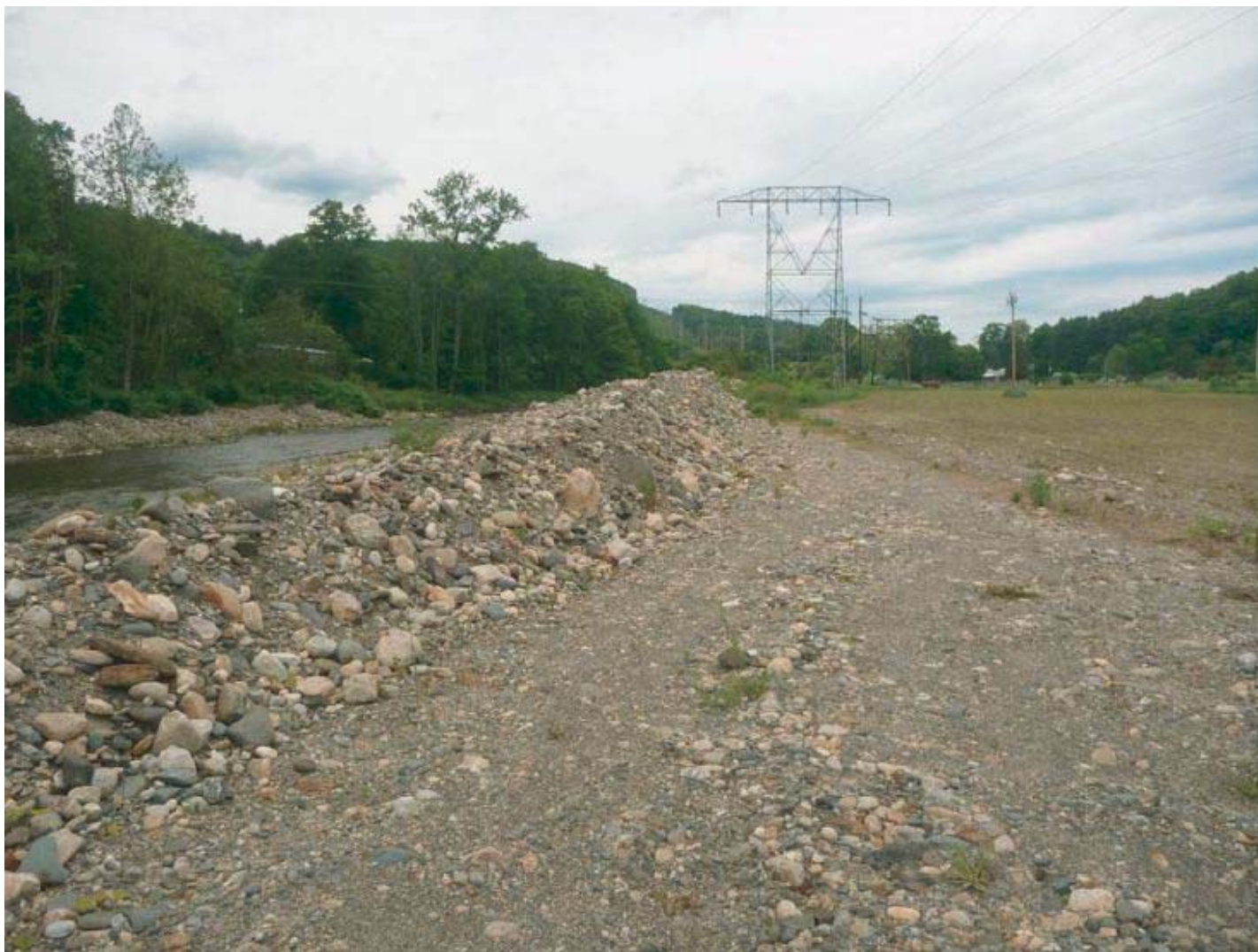
Figure 6. A berm built on the bank of the West Branch of North River as part of the post-Irene emergency work.
