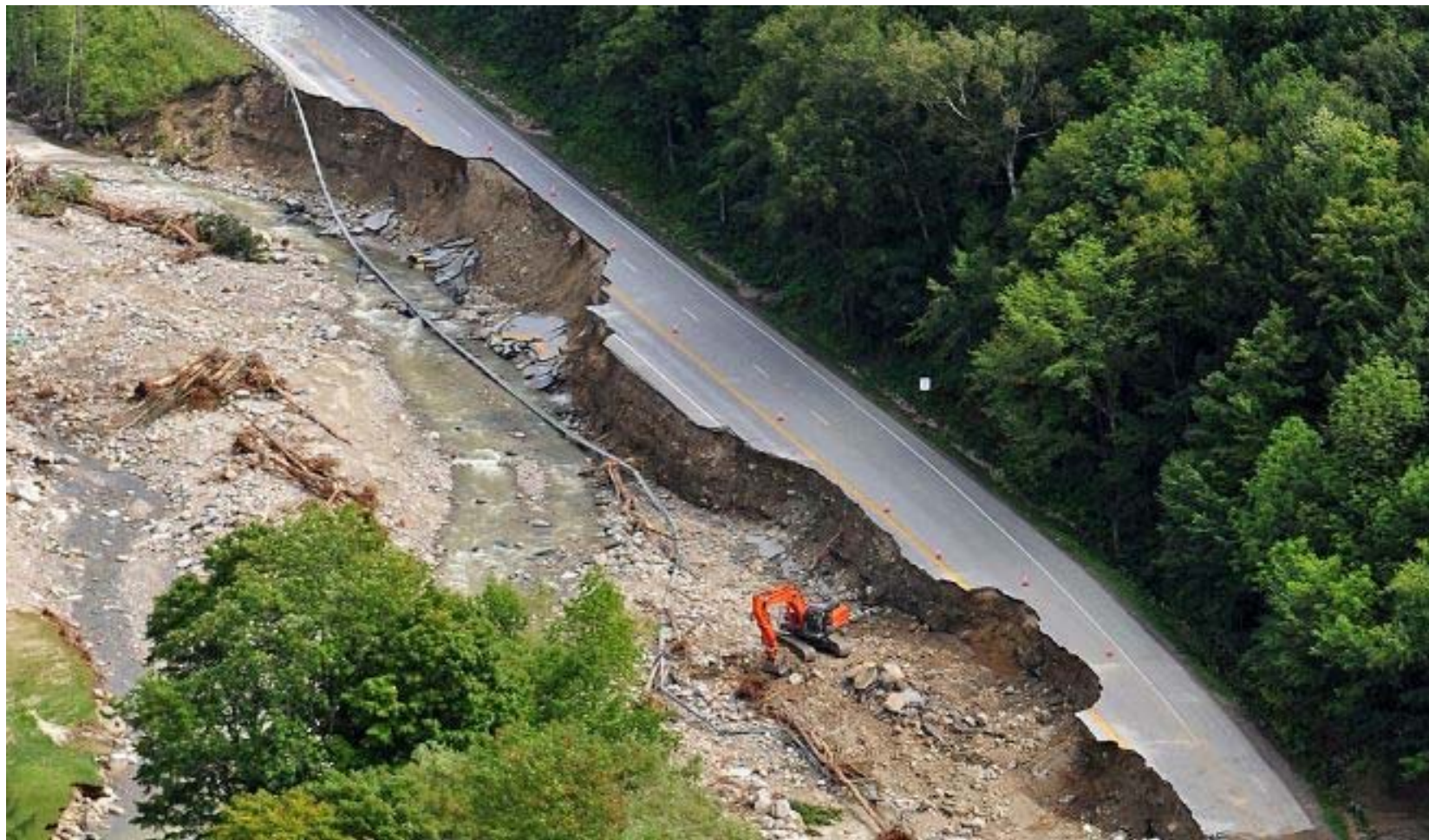
Figure 3. Significant recession of an elevated river terrace occurred in Mendon, VT during Tropical Storm Irene washing out portions of Route 4.
