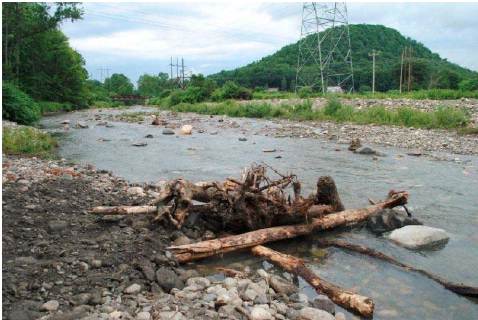
Figure 7. Wood and boulders added to the West Branch channel as part of restoration efforts following Tropical Storm Irene and post-flood emergency work.
