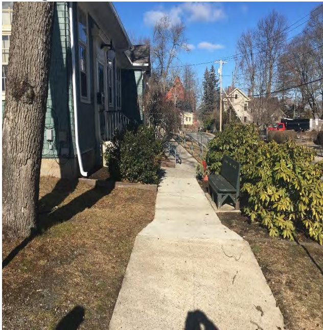
"Before Picture" showing cracks on bumpy unleveled sidewalk
