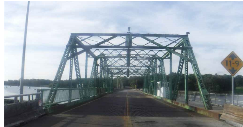
Kernwood Avenue Bridge, connecting Beverly and Salem
