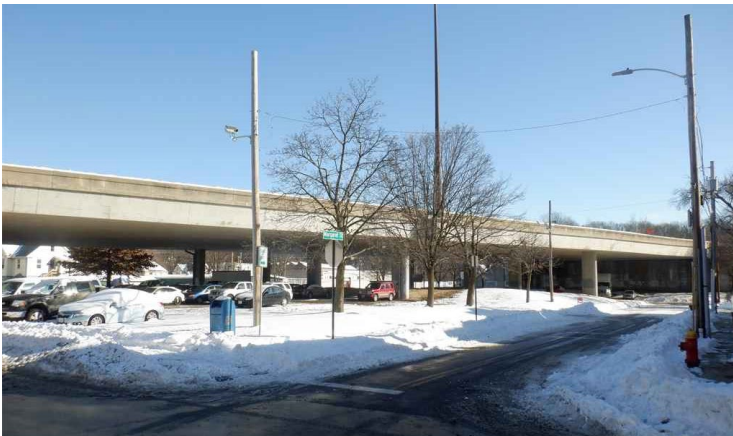
I-391 Bridge over Route 116, Chicopee
