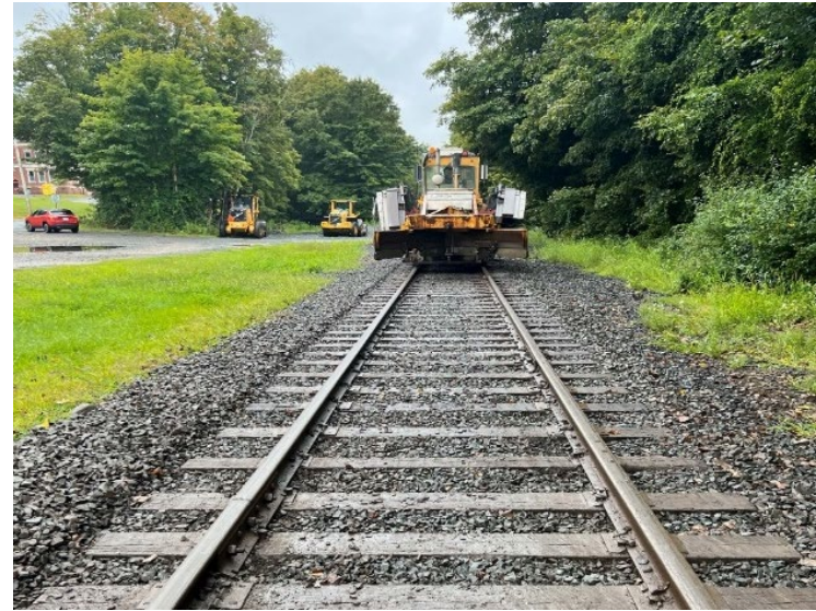
Ballast regulator operation on rail line
