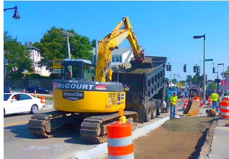
Roadway construction equipment
