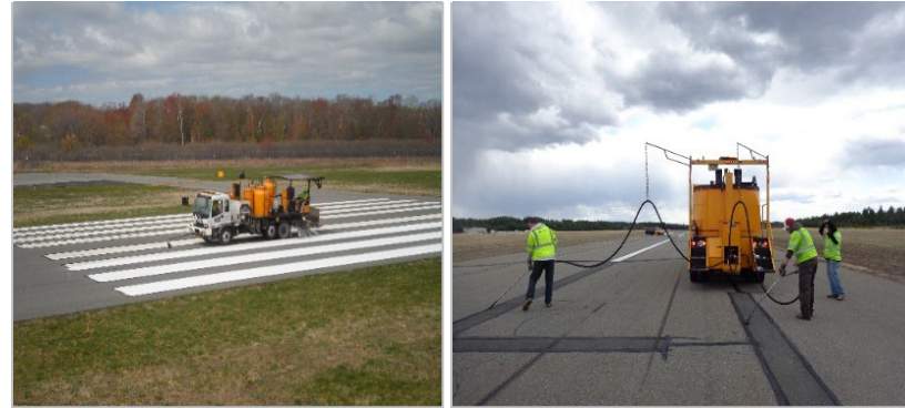
Statewide deck sealing and airfield marking projects
