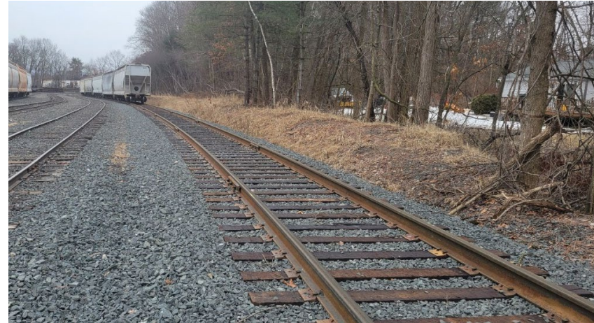
Pioneer Valley Railroad, Easthampton Yard track
