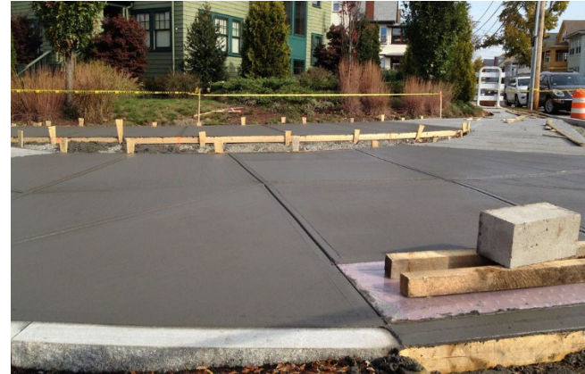
Curb cut improvements
