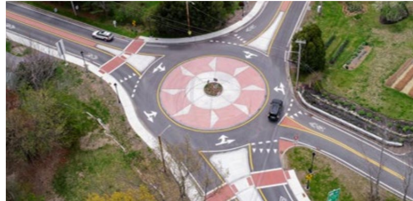
Roundabout on Route 140, Princeton
