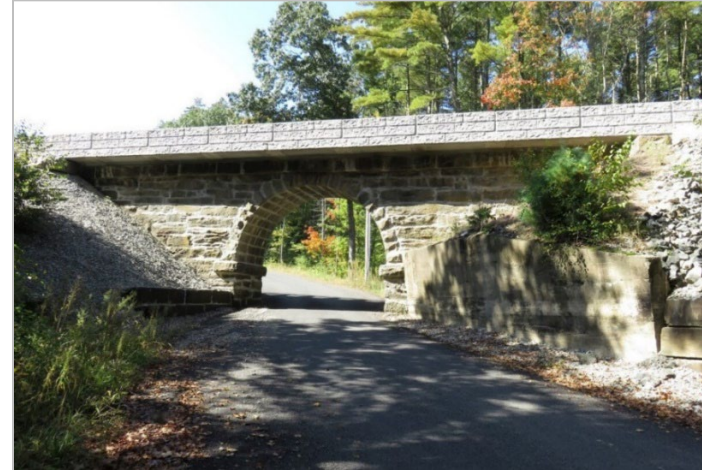
Rail bridge arch deck concrete repair
