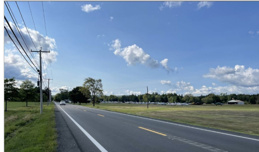
Pavement improvements in Great Barrington
