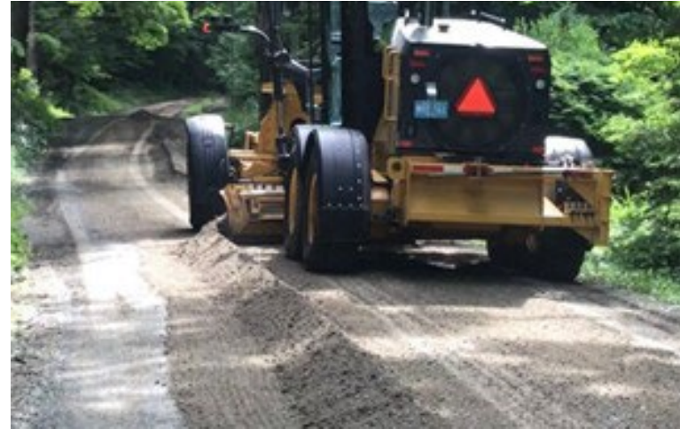
Example of unpaved road
