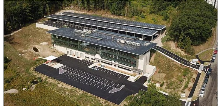
MassDOT Highway District 3 Office
