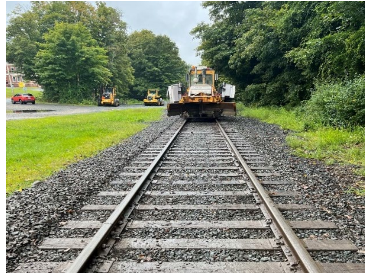
Ballast regulator operation on rail line
