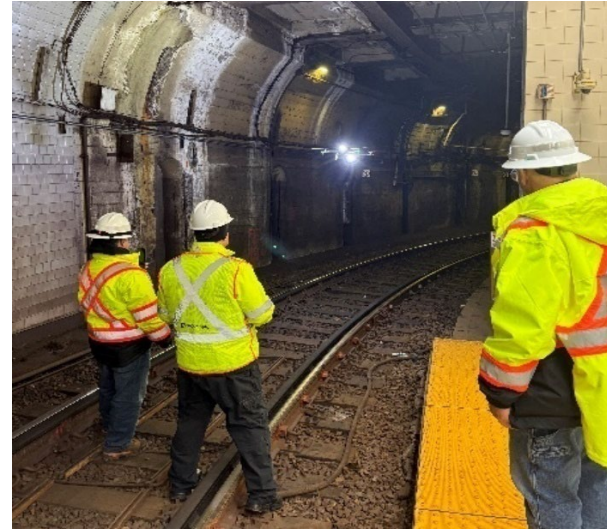
Team performing tunnel inspection using drones
