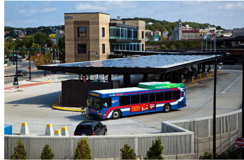
Union Station Bus Transfer Facility in Worcester
