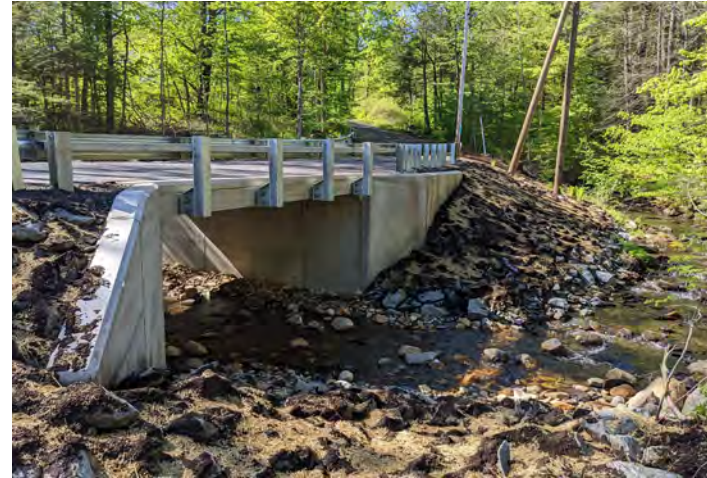
Example of small bridges
