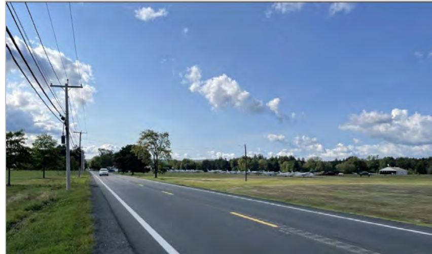
Pavement improvements in Great Barrington
