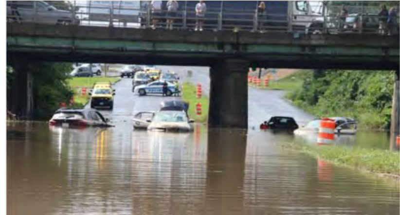
Resilience project location –Route 20/ Route 122 interchange, Worcester
