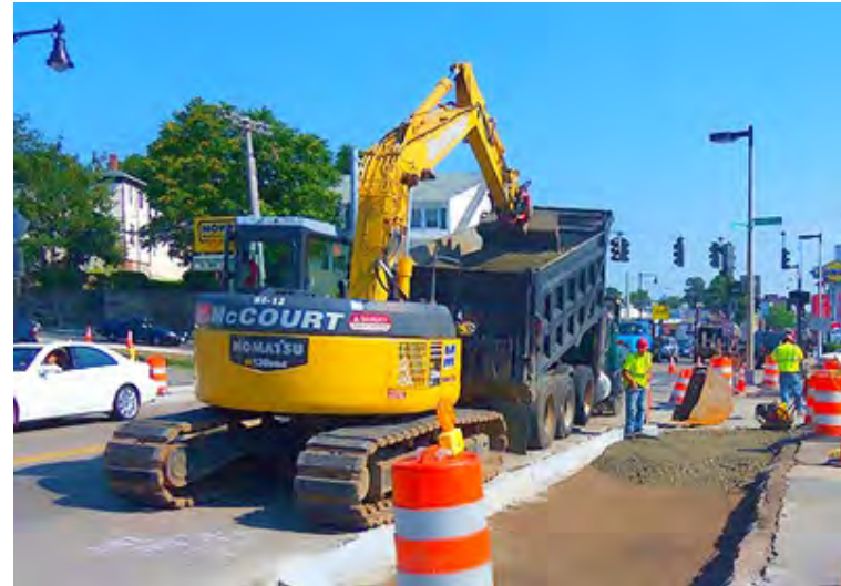
Roadway construction equipment
