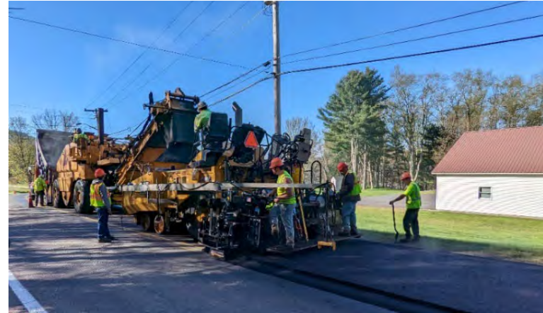
Paving equipment and crew on a local roadway
