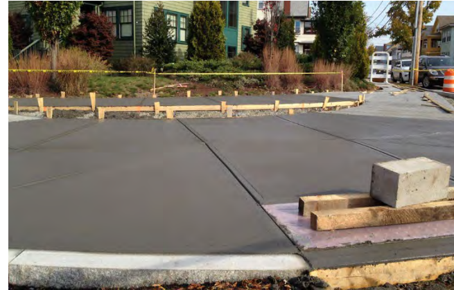
Curb cut improvements
