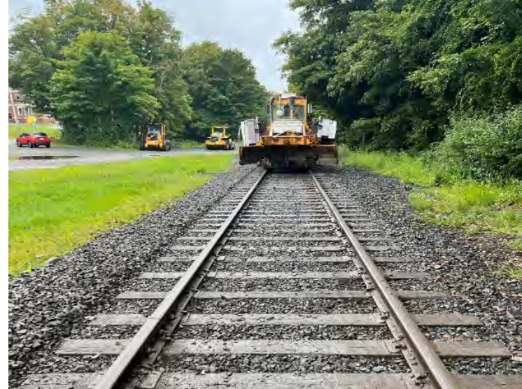
Ballast regulator operation on rail line
