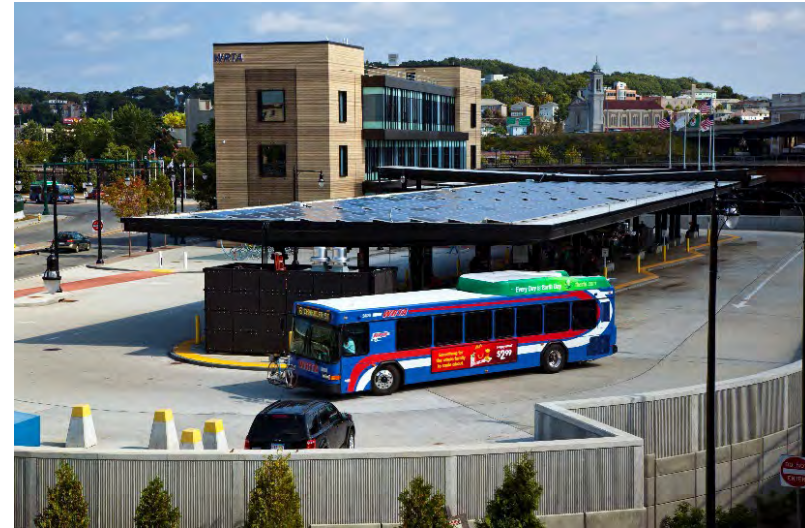
Union Station Bus Transfer Facility in Worcester
