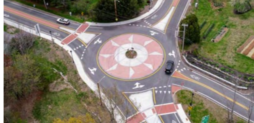
Roundabout on Route 140, Princeton
