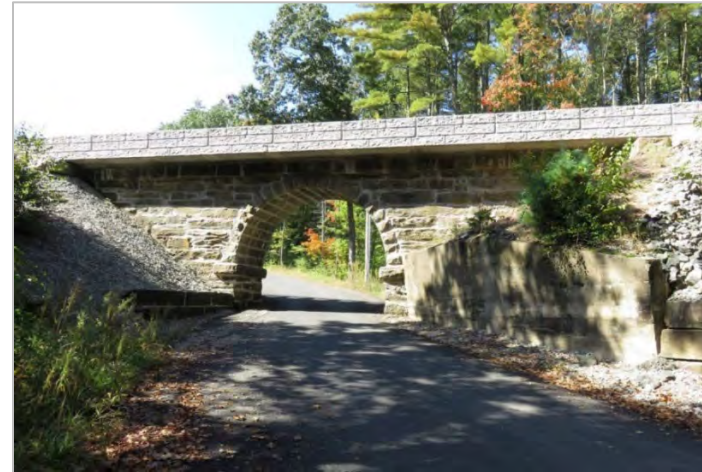
Rail bridge arch deck concrete repair
