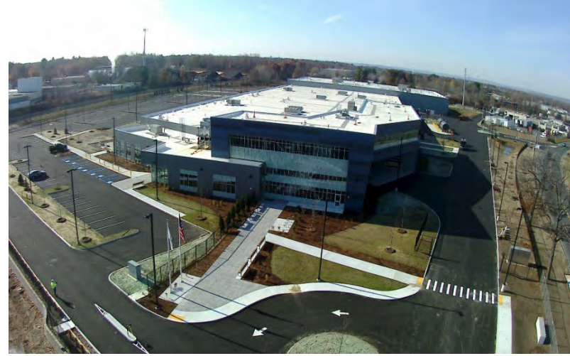
Pioneer Valley Transit Authority Maintenance Facility
