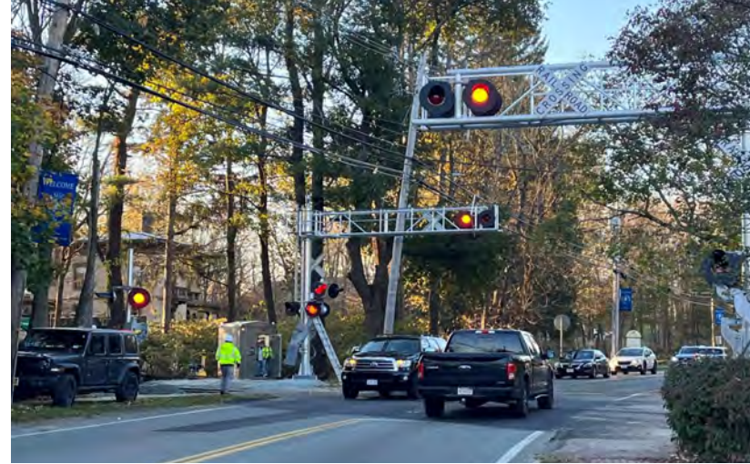
Crossing signal upgrades in Sherborn
