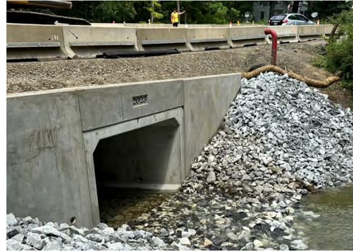
New Box Culvert installed on Route 23 in Egremont
