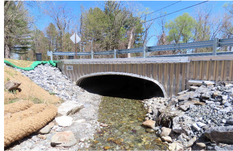
Elevation culvert in Richmond
