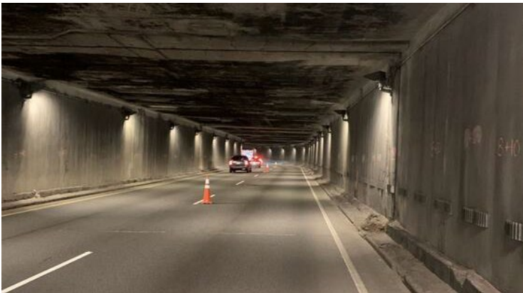
Storrow Drive Tunnel interior
