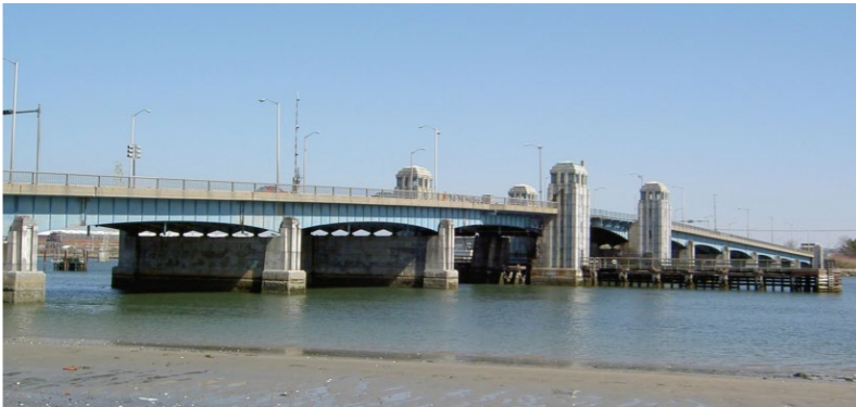
General Edwards Bridge in Lynn
