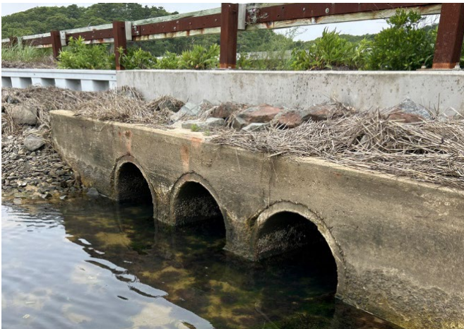
Completed culvert project on Route 6 in Provincetown
