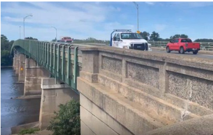
US 20 over Connecticut River, connecting Springfield and West Springfield
