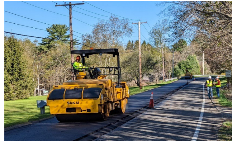
Paving equipment on local roadways
