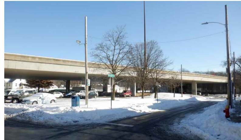
I-391 Bridge over Route 116, Chicopee
