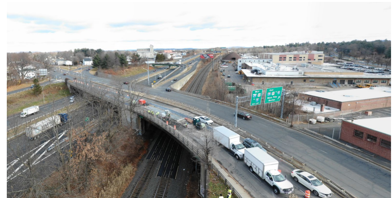
St James Avenue Bridge over I-291 and CSX Railroad
