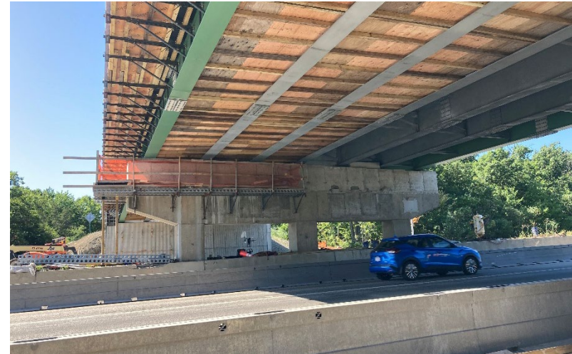
Bridge preservation work in Millbury
