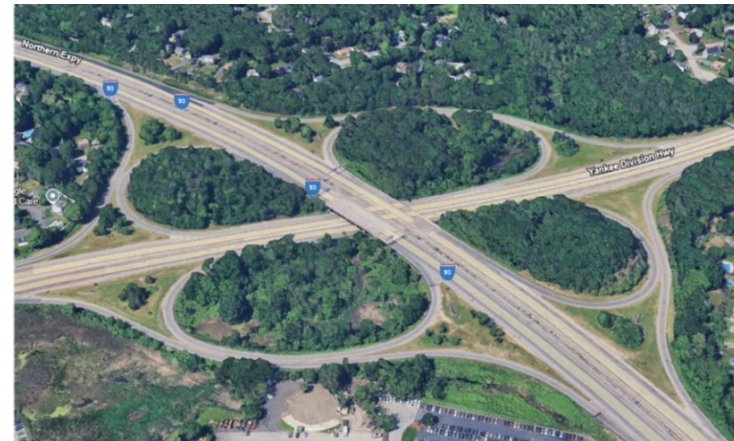
I-93/I-95 Interchange Improvements in Woburn and Reading
