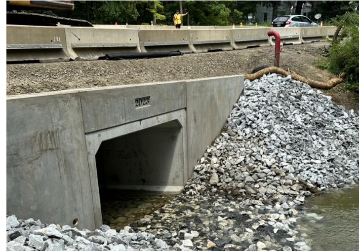
Example culvert improvement project in Egremont
