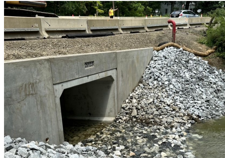
Example culvert improvement project in Egremont
