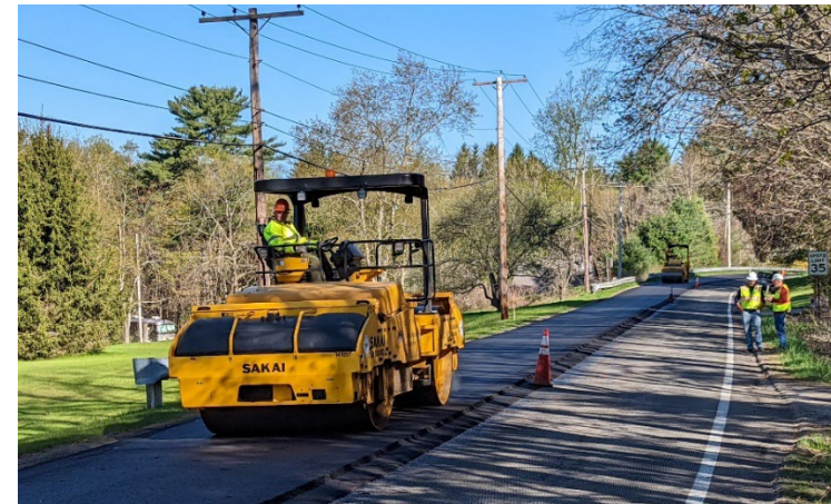
Paving equipment on local roadways
