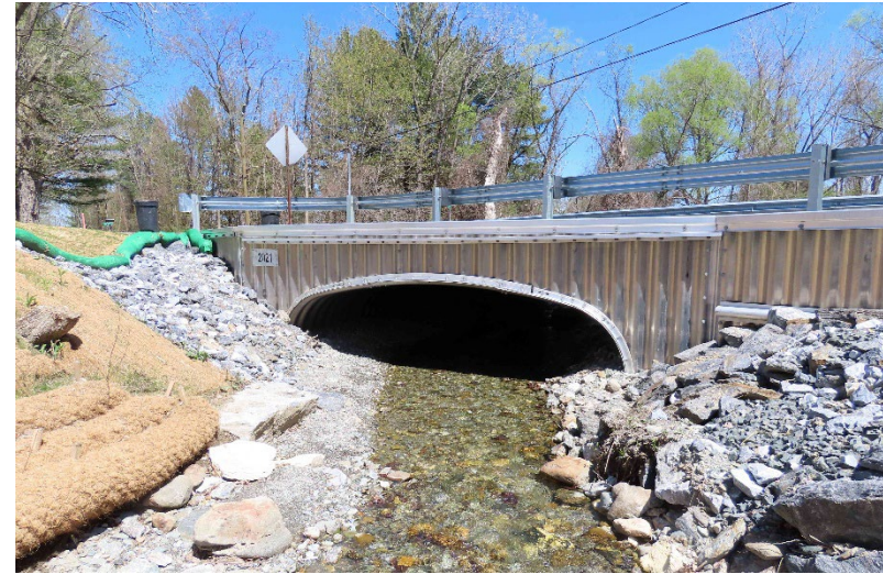
Elevation culvert in Richmond
