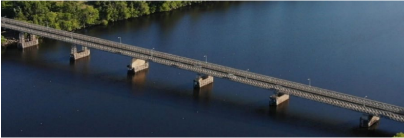
Rourke Bridge in Lowell
