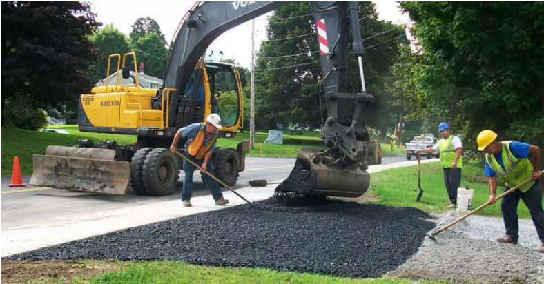
Roadway repaving project
