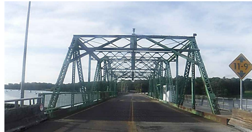
Kernwood Avenue Bridge, connecting Beverly and Salem
