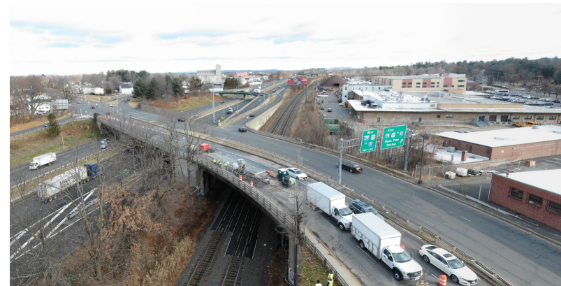
St James Avenue Bridge over I-291 and CSX Railroad
