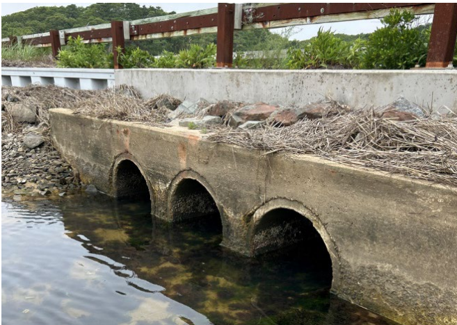
Completed culvert project on Route 6 in Provincetown
