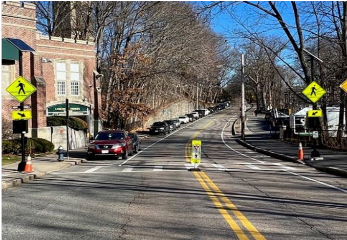
Pedestrian crossing improvement project in Brookline
