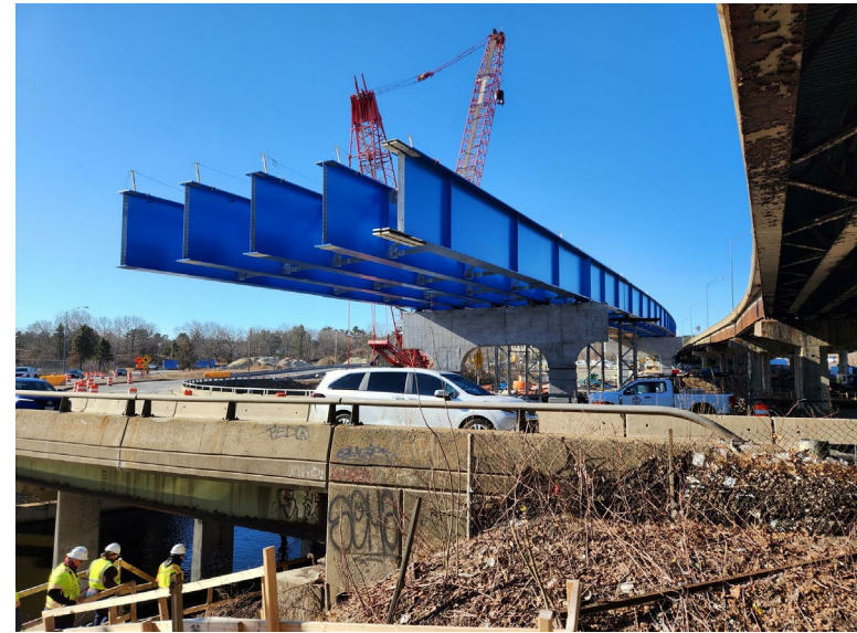
Newton & Weston – I-90 / I-95 interchange construction
