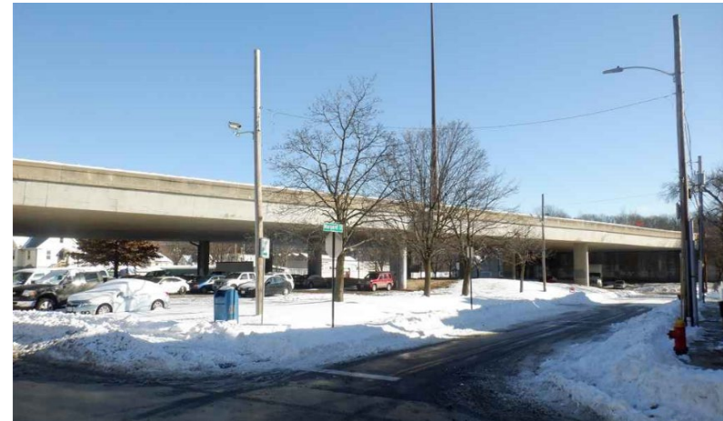
I-391 Bridge over Route 116, Chicopee
