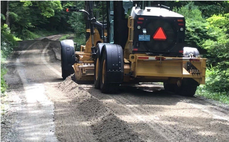
Roadwork on unpaved road
