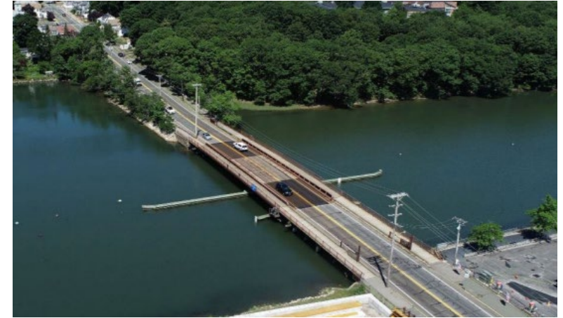
Existing Hall-Whitaker bridge in Beverly
