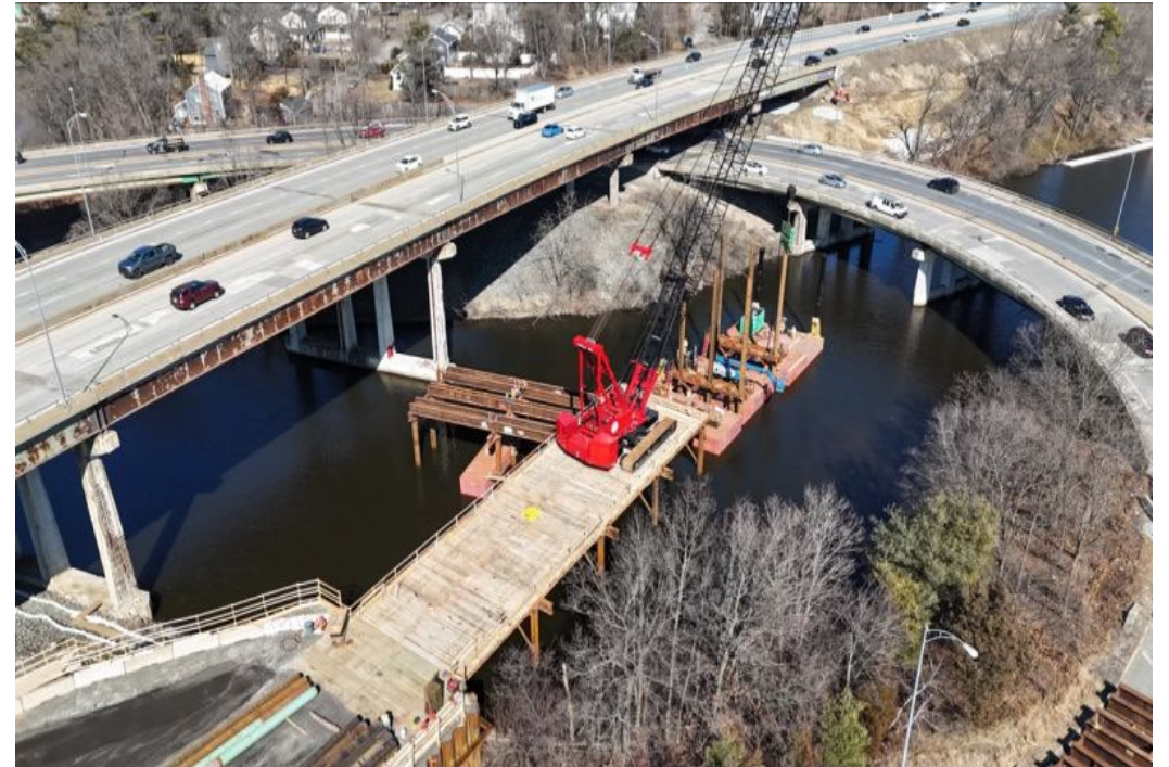
Newton-Weston Bridge Construction
