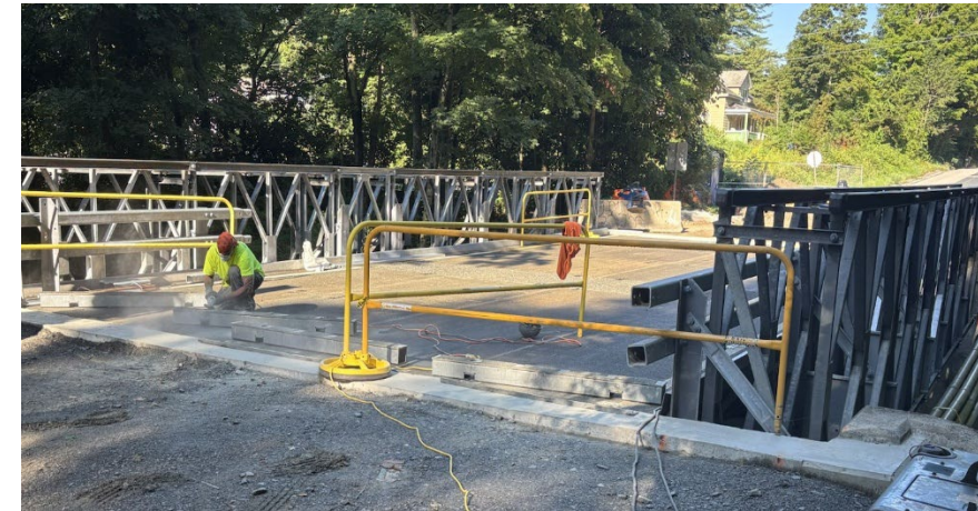
Above: Installation of temporary bridge in Dudley
