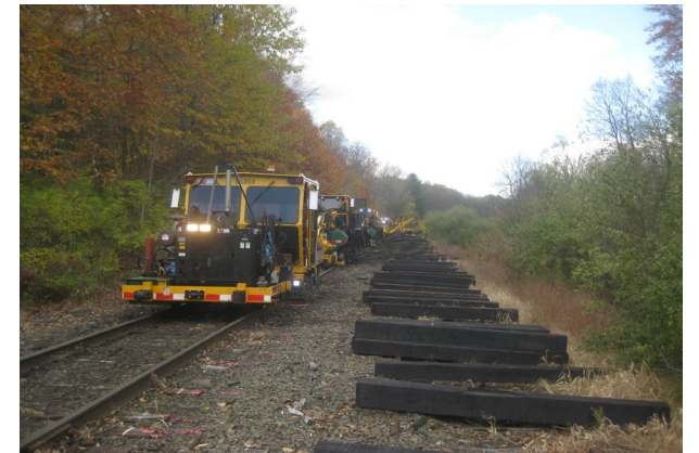
Above: Railworks Tie Gang, Pittsfield – Berkshire Line Tie Project
