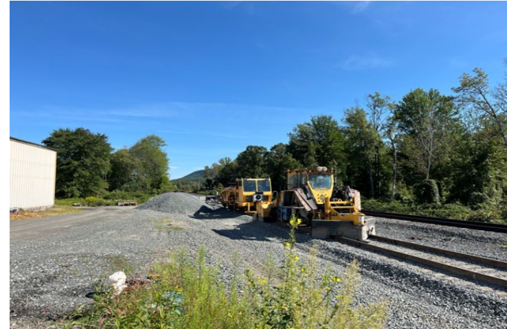
Left: Deerfield MOW Siding Installation
