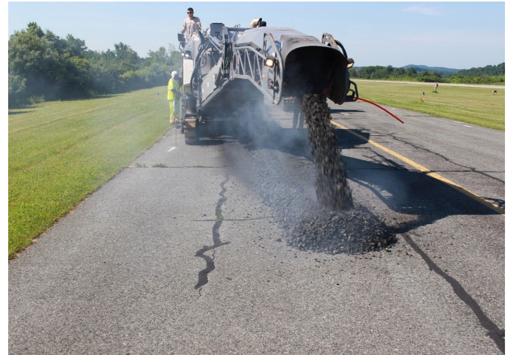
Above: Aeronautics Pavement Maintenance Operations
