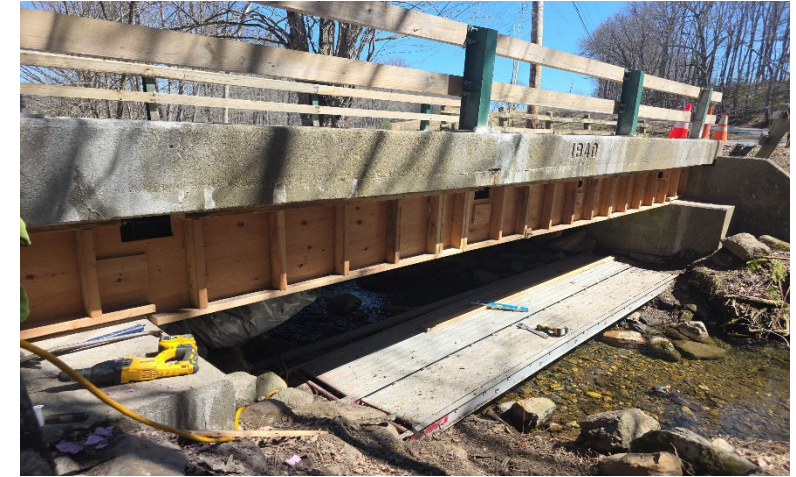
Left: Beam Repairs over Water Bear River Bridge in Ashfield
