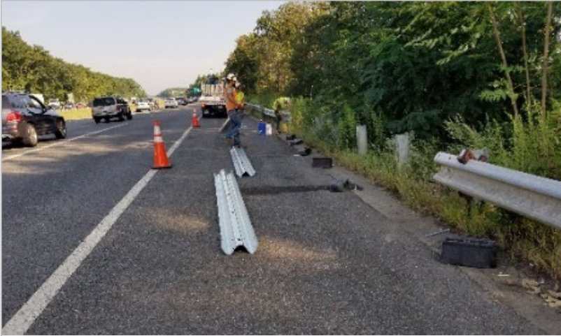
Guard rail improvements
