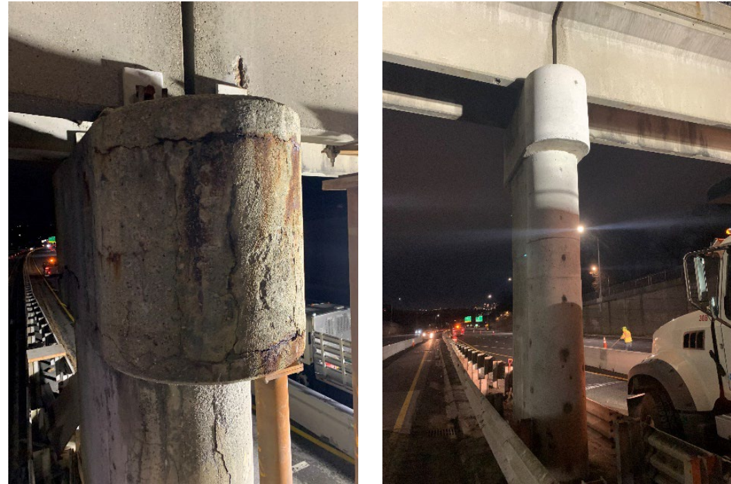
Before/After, repair of pier supporting pedestrian bridge over route 2, Arlington
