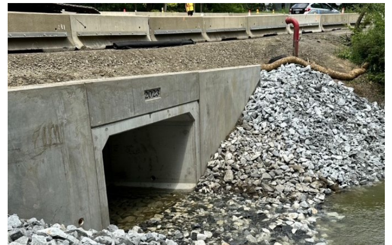
New box culvert on Route 23 in Egremont
