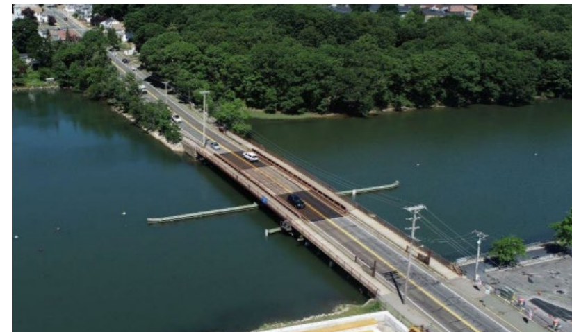
Existing Hall-Whitaker bridge in Beverly
