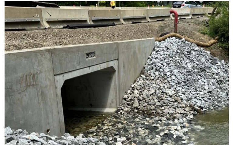
New box culvert on Route 23 in Egremont
