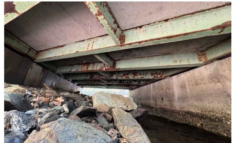
Posted bridge on Route 183 in Sandisfield
