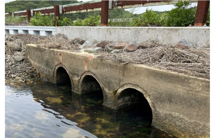
Completed culvert project on Route 6 in Provincetown
