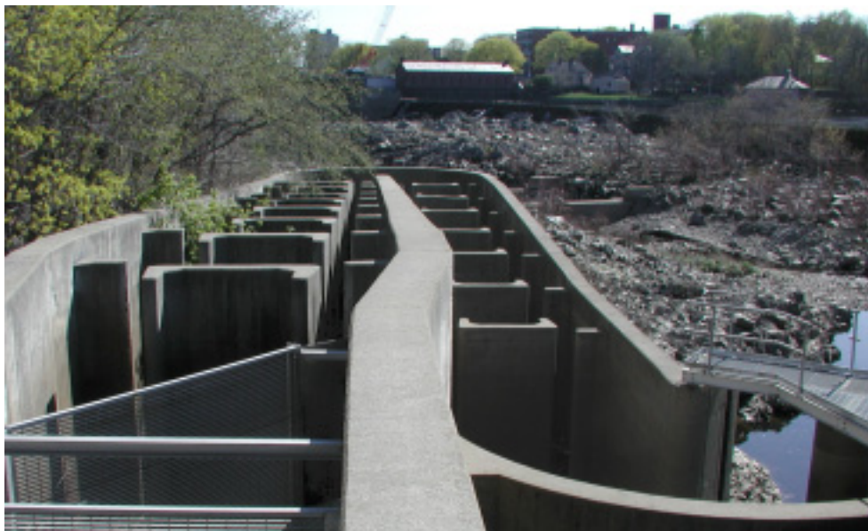
Modified Ice Harbor vertical slot fishway – Pawtucket Dam, Lowell
