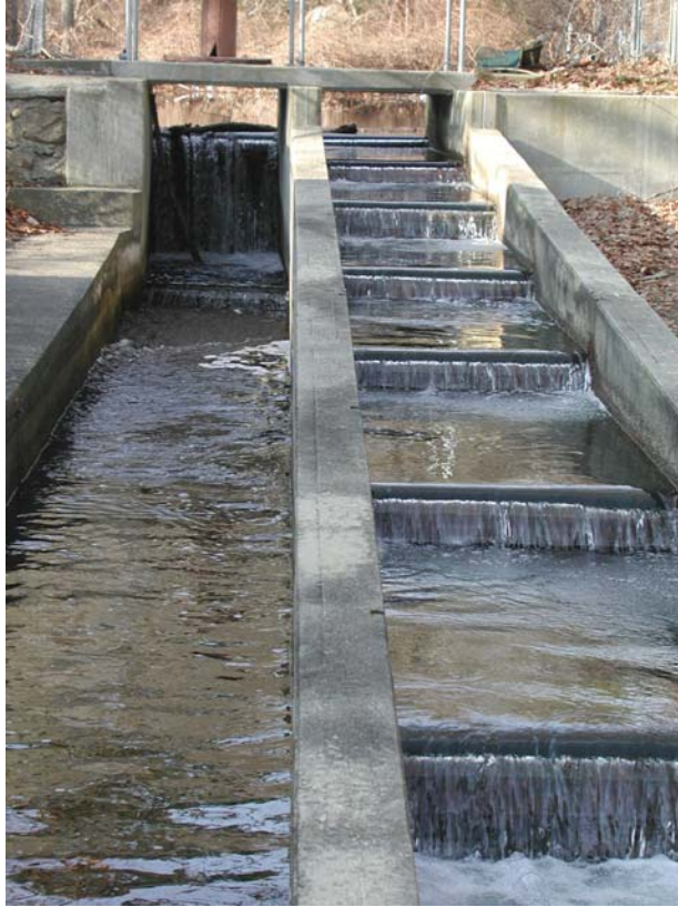
Weir pool – Benoit's Pond Dam, Bourne
