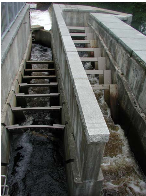
Denil – Newton Lower Falls, Newton
