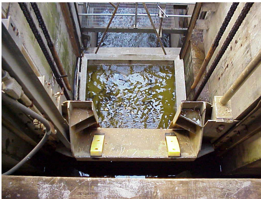
Fish lift – hopper rising with fish –Essex Dam, Lawrence
