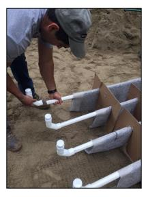
This distribution pipe, with or without the extension pipe, should pitch back to the GeoMat to prevent freezing.
