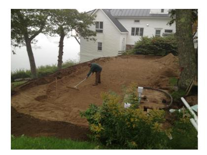
summary, uniform sand density is critical to system performance and can be negatively impacted by machinery and other static and dynamic loads on the sand base.
