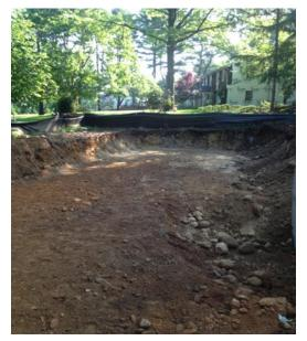
entire leach field area may be excavated as necessary and backfilled with a minimum 6 inch layer of approved sand to the design elevation.
