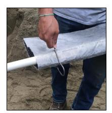
**10.2.5.** Fasten pipe into place inside the GeoMat with Geomatrix stake clips on approximately 24 inch centers.
