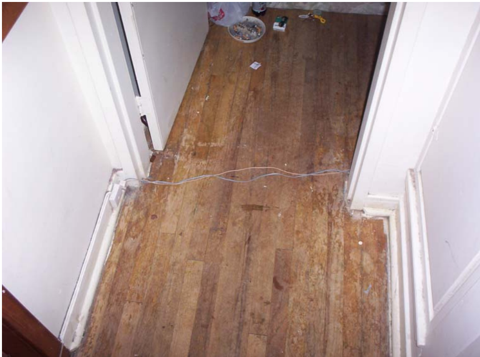
200-1 Development, 70 Veterans Way Temporary Wiring on Bedroom and Living Room Floor
