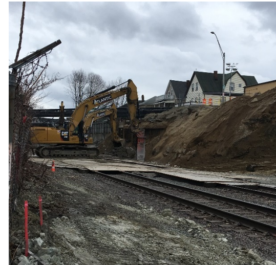
West Abutment Demolition
