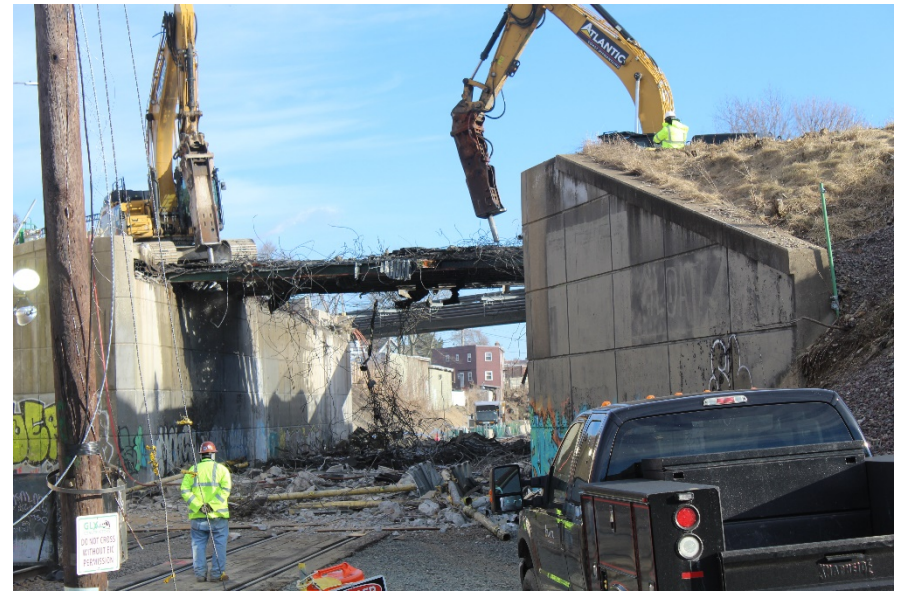
Superstructure Removal
